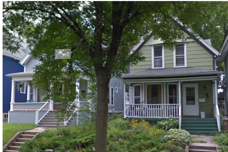
Front Porch on House with Nonconforming Side Yard Setback
