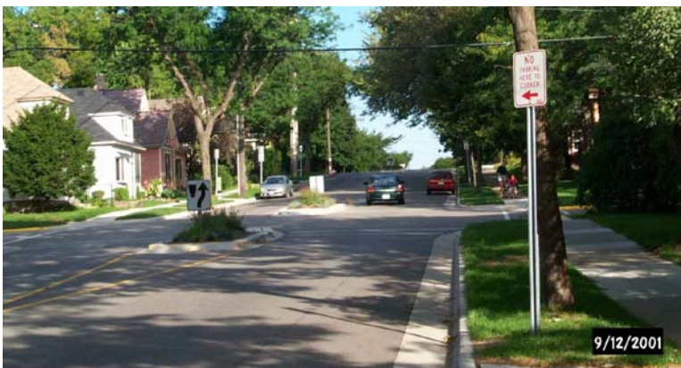
Typical parking restriction for a pedestrian refuge island (N. Baldwin St. at Mifflin St)
