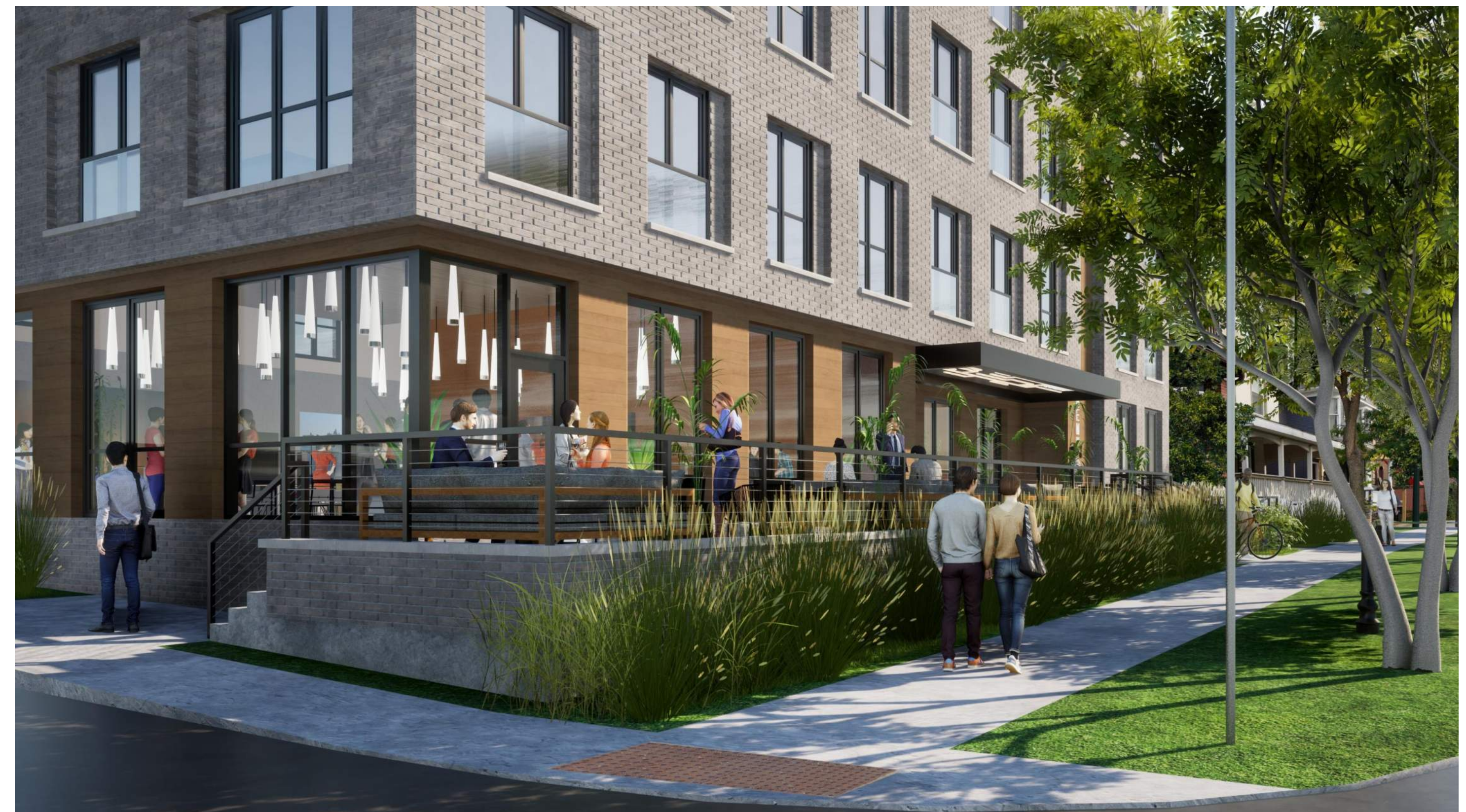
Looking Southeast from corner of Mendota Ct and N Lake St
