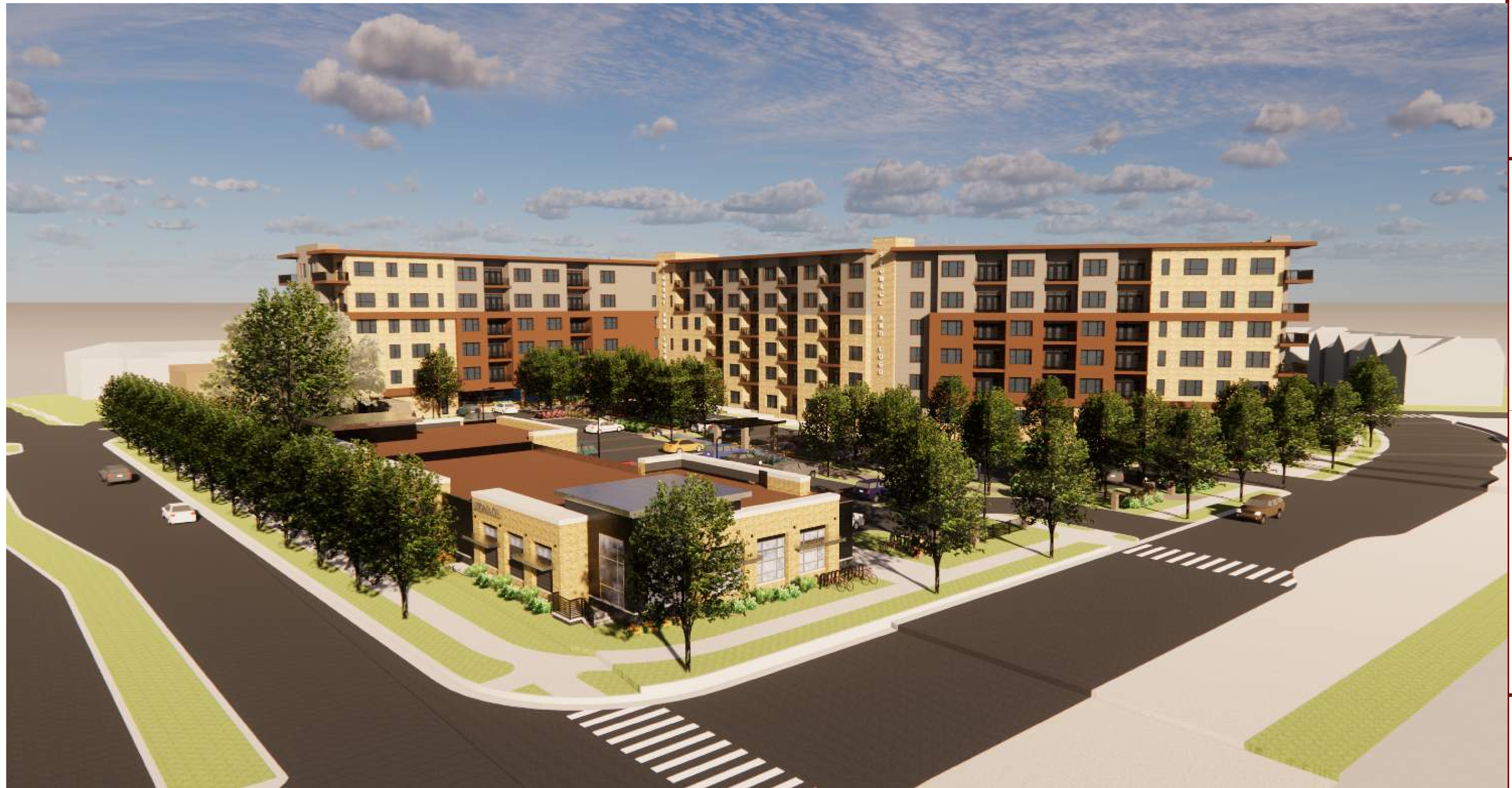
VIEW FROM COTTAGE GROVE ROAD & GEMINI DRIVE
