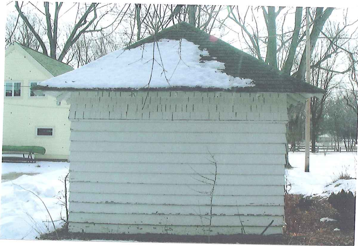
EXISTING SHED (TO BE DEMOLISHED)
