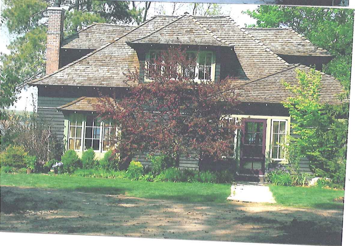
EXISTING RESIDENCE (AFTER RENOVATIONS)
