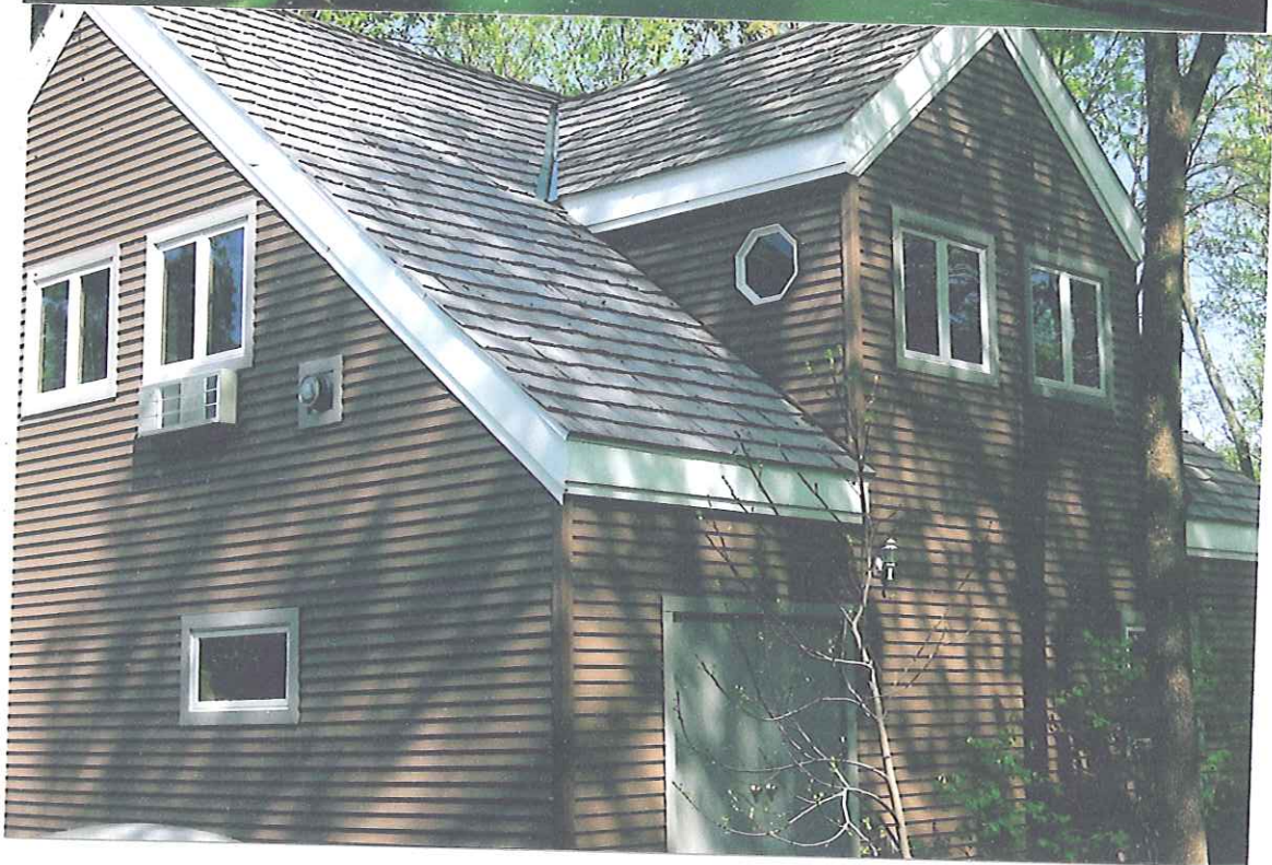
GARAGE / CARRIAGE HOUSE NEXT DOOR (5620 LAKE MENDOTA DR)
