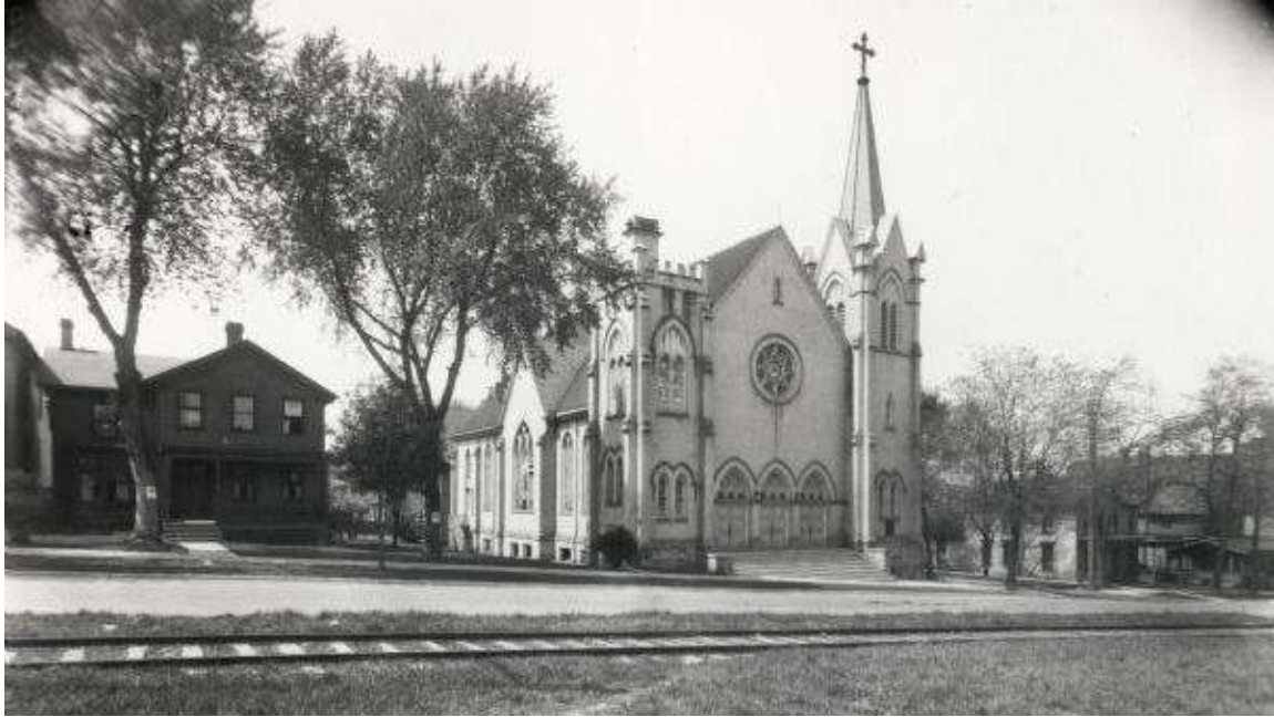
Photograph of St. John's Lutheran Church taken from the south, 1918. On file at the Wisconsin Historical Society Library and Archives. The house across Hancock Street on the left side of the photo are the subjects of this report.
