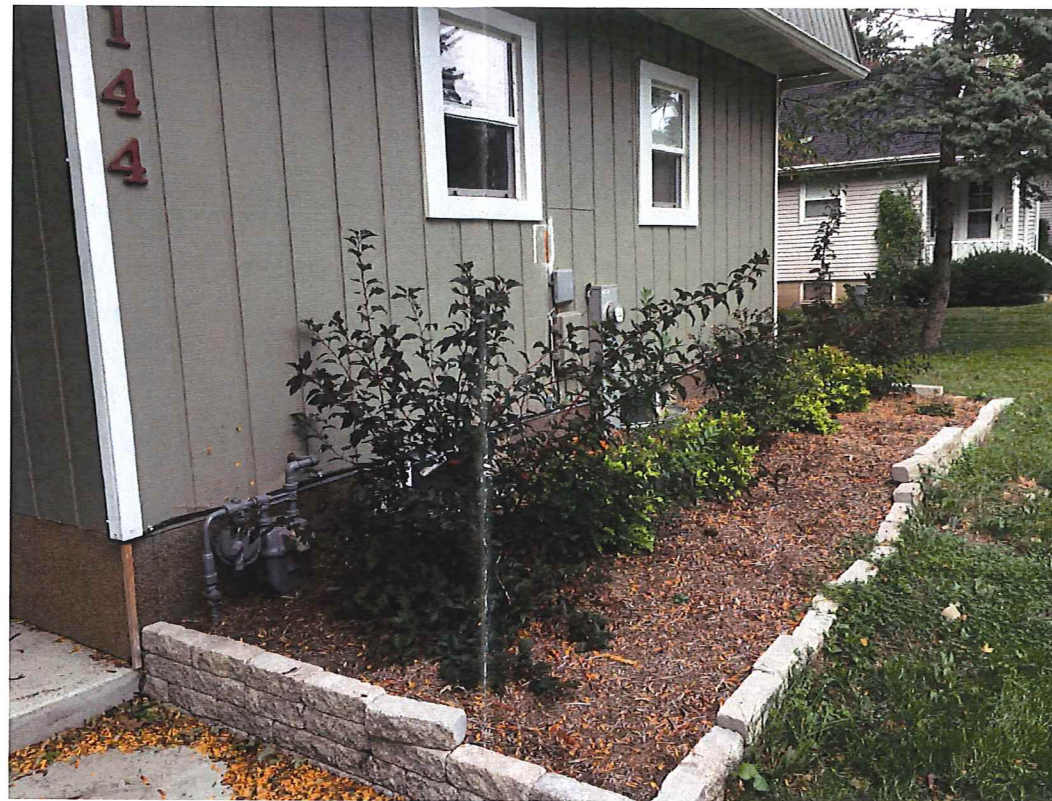
Photo of affected area in front of house
