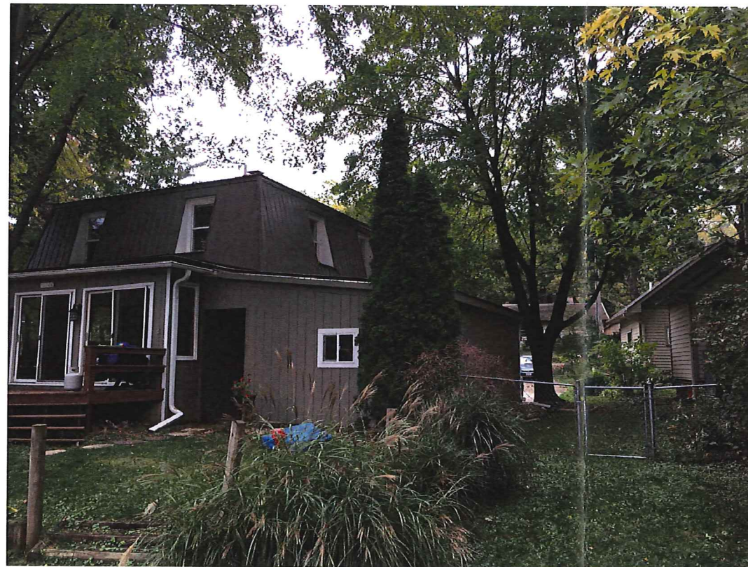
Photo of affected area in rear of house
