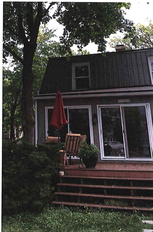
Photo of existing north east corner
