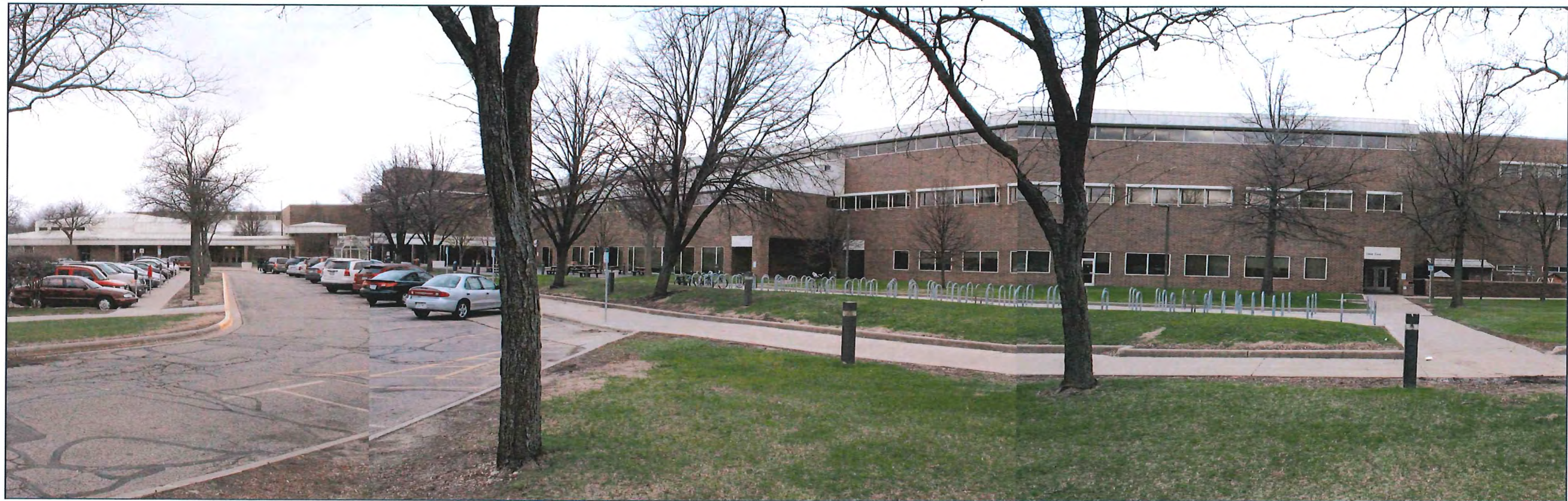
EXISTING ADMINISTRATION BUILDING ENTRY
