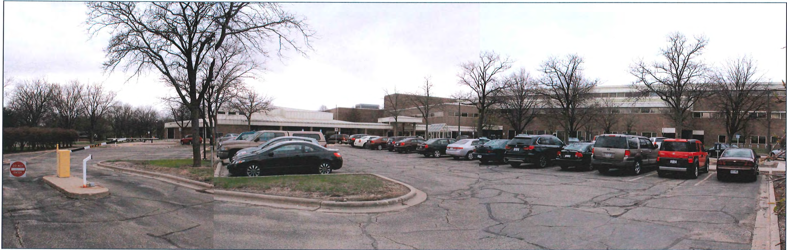
EXISTING ADMINISTRATION BUILDING ENTRY
