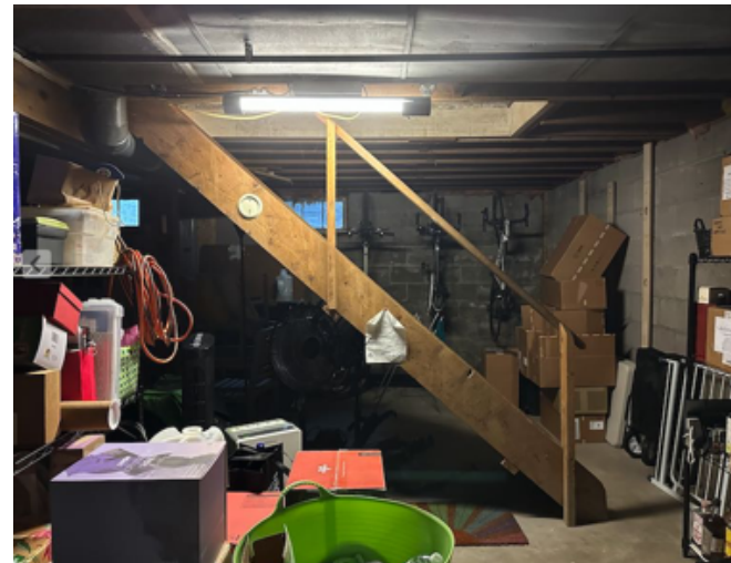
the first floor is framed with 2x8 joists set directly on the concrete with no treated wood sill plate. the ductwork is in need of replacement . there is single undersized central return and one upstairs bedroom has no registers.
