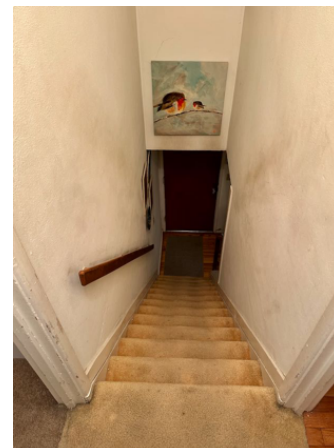
staircase 2'-7" wide with 7" deep treads
