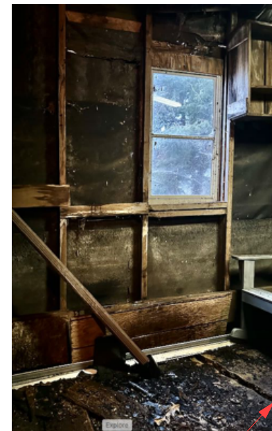
garage interior large crack in slab holes in roofing structure is rotten
