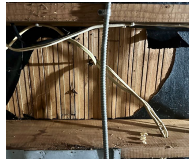
the house has no subflooring. the wood T&G boards are installed directly to the floor joists
