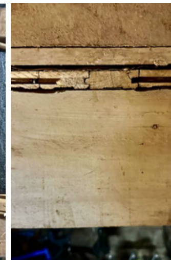
the house has no subflooring. the wood T&G boards are installed directly to the floor joists
