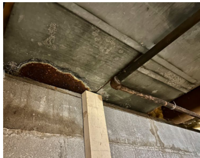
the first floor is framed with 2x8 joists set directly on the concrete with no treated wood sill plate. the ductwork is in need of replacement . there is single undersized central return and one upstairs bedroom has no registers.
