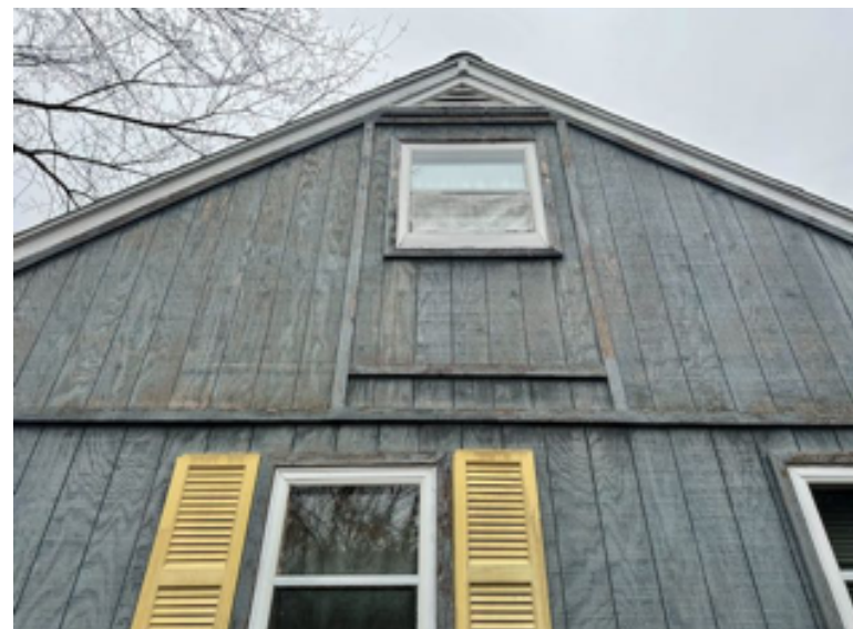
typical condition of windows and trim
