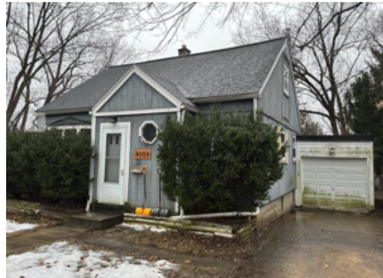
front/ west side view
