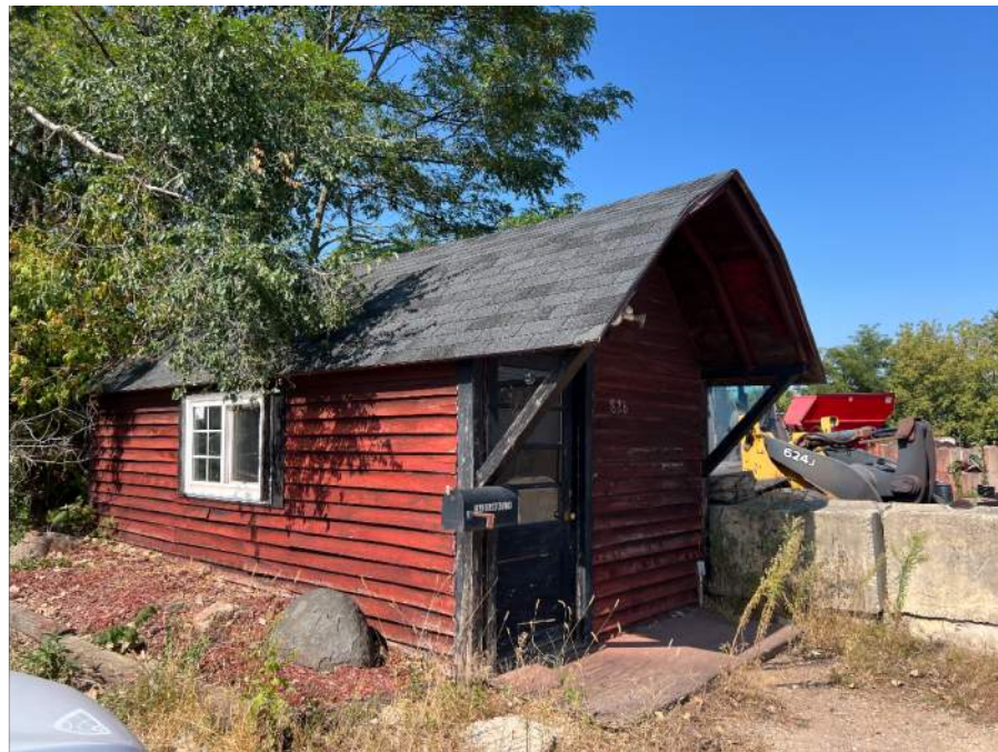
826 NORTH AVE - SHED
