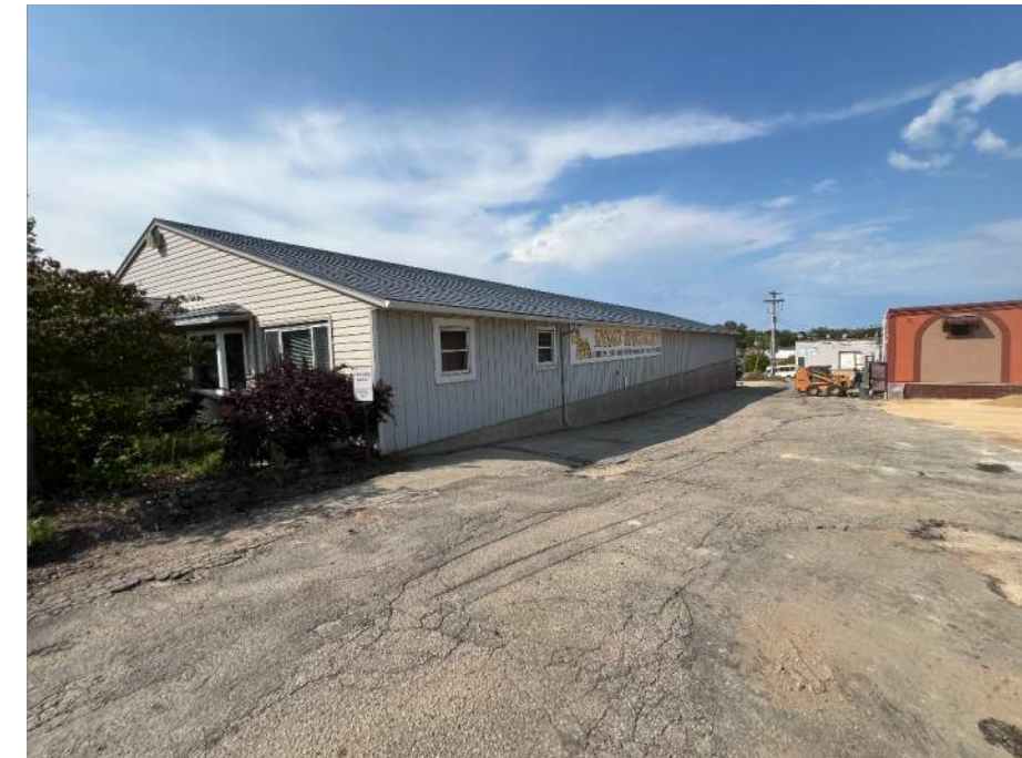
814 NORTH AVE - VIEW OF EAST WALL FROM NORTH AVE
