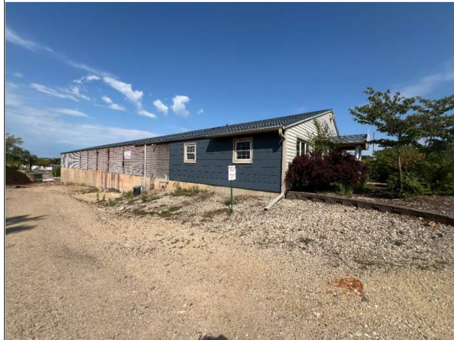
814 NORTH AVE - VIEW OF WEST WALL
