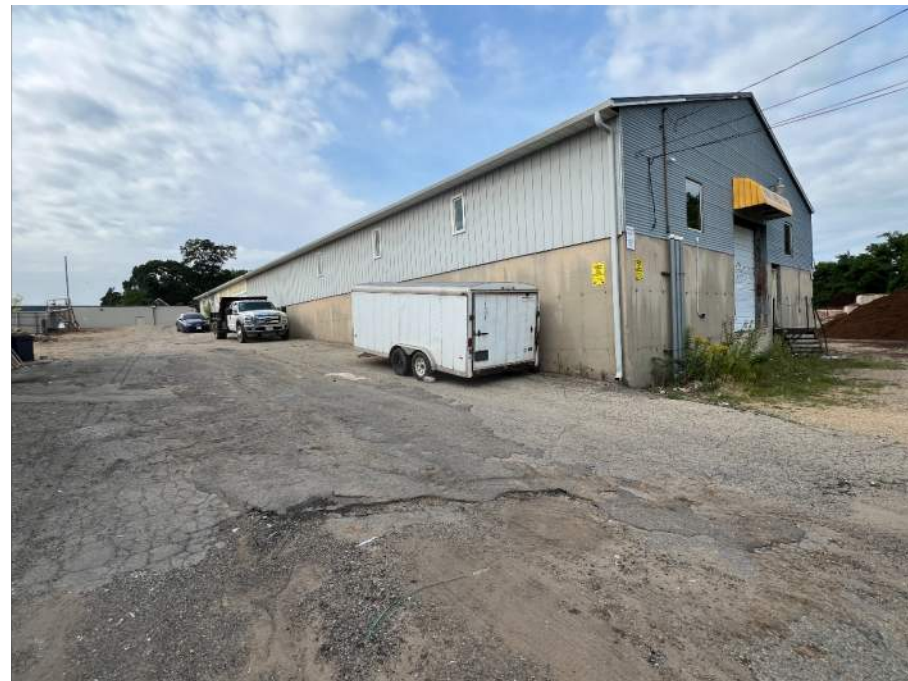
814 NORTH AVE - VIEW OF REAR AND EAST WALL
