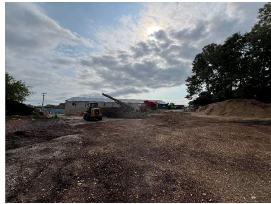
826 NORTH AVE - LOOKING EAST TOWARDS 814 NORTH AVE.
