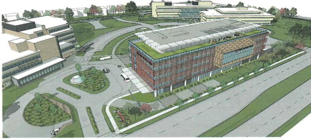
AERIAL VIEW FROM SOUTHWEST, OVER MINERAL POINT ROAD
