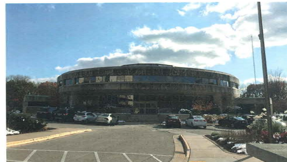
EXISTING VIEW FROM PARKING LOT, NORTH ELEVATION
