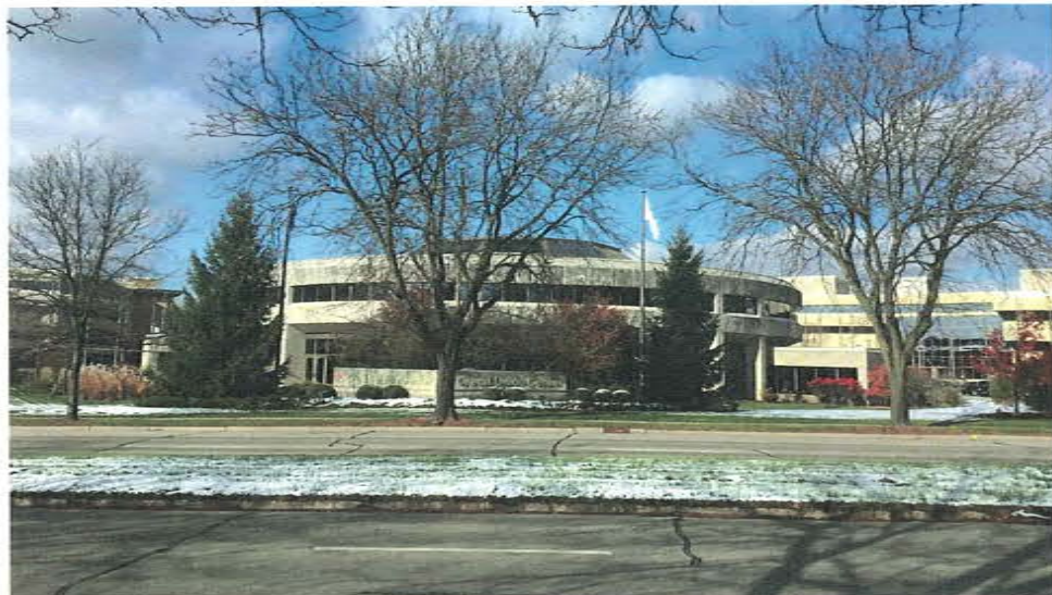
EXISTING VIEW FROM MINERAL POINT ROAD, SOUTH ELEVATION
