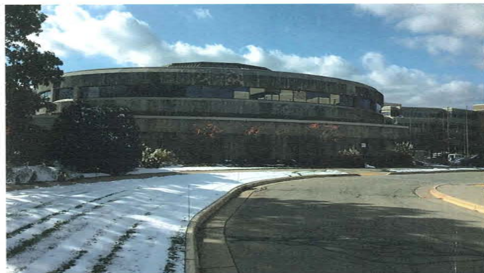
EXISTING VIEW FROM DRIVEWAY OFF MINERAL POINT ROAD, EAST ELEVATION
