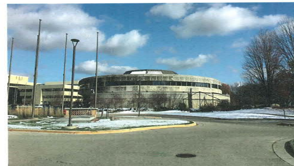
EXISTING VIEW FROM PARKING LOT, SOUTHWEST ELEVATION
