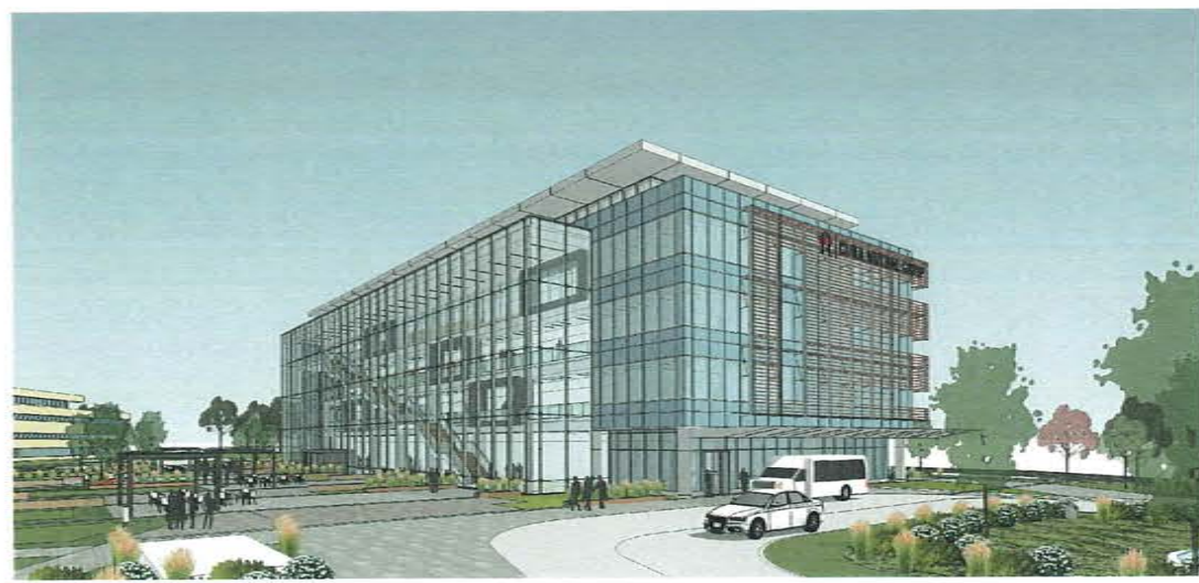
VIEW OF NEW 5810 ENTRY FROM 5910 BUILDING
