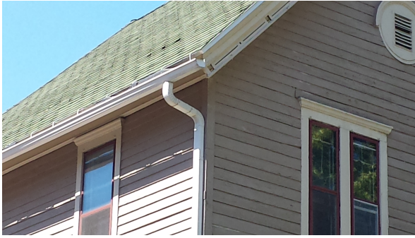
K Gutters on 18 W. Gilman
