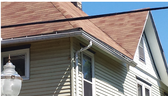
K Gutters on 21 W. Gilman
