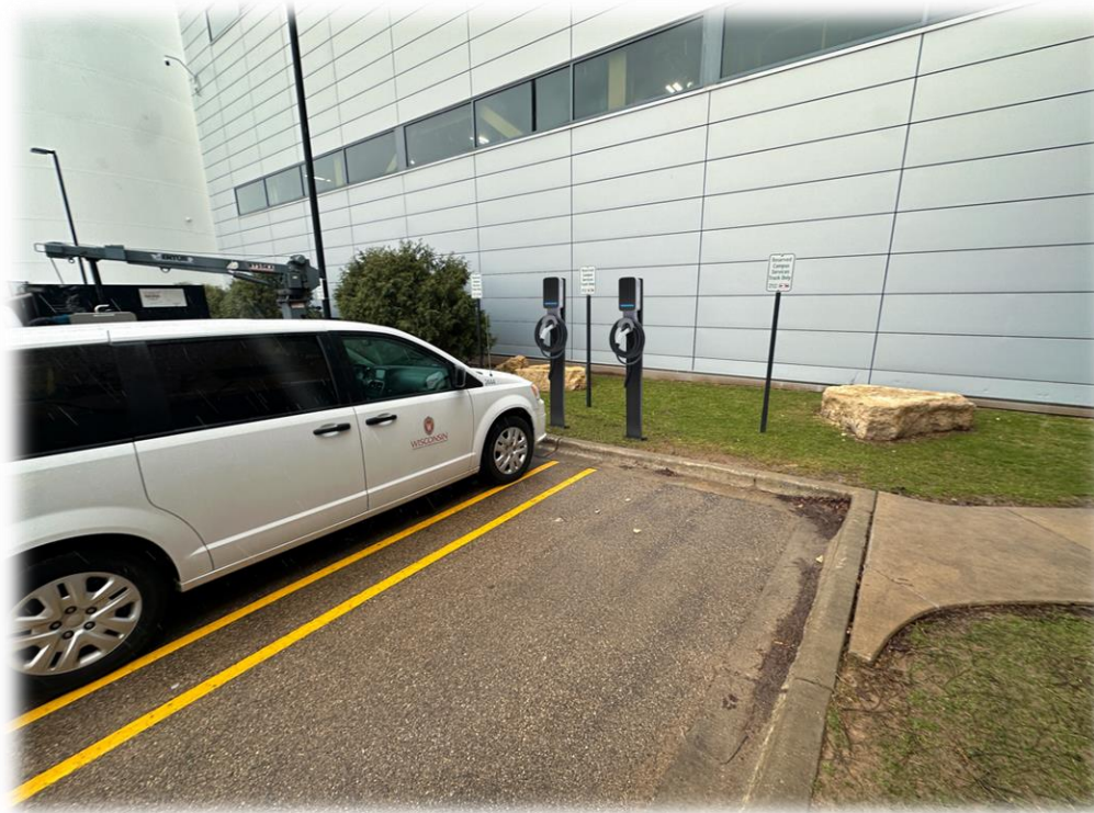
Lot 33 - Charter Steet Heating Plant
