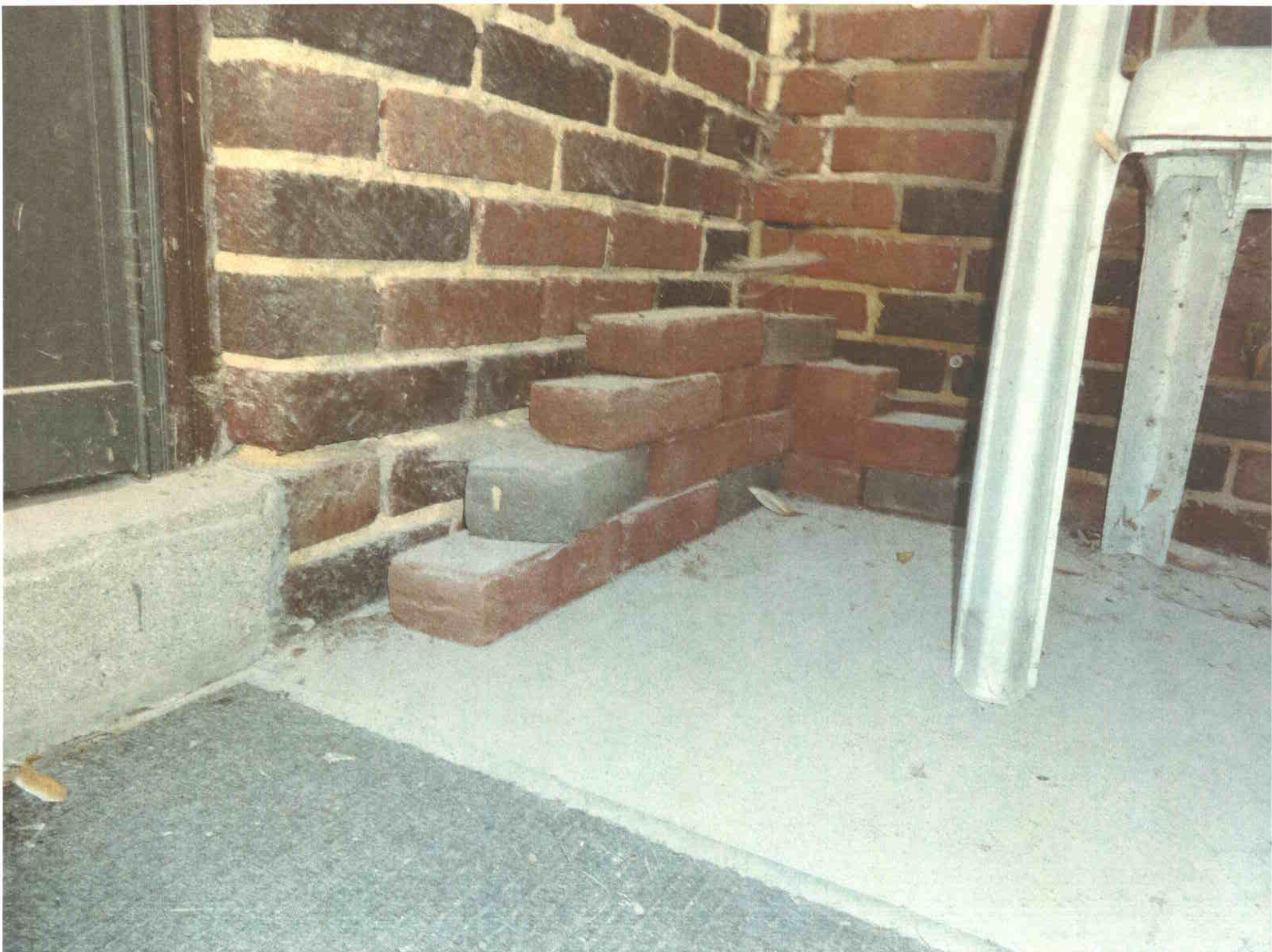
8-28-2013 SAMPLE OF NEW BRICKS TO MATCH EXISTING
