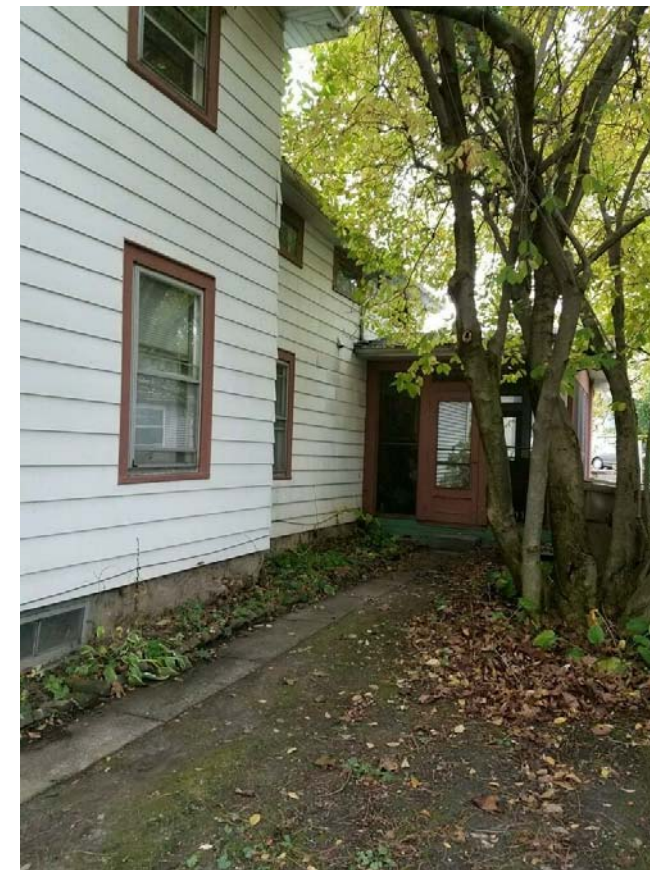
921 WEST SIDE YARD - PRIOR TO DEMO
