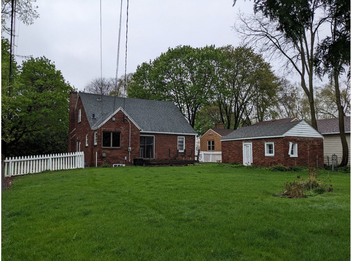
East Rear Elevation and Shed
