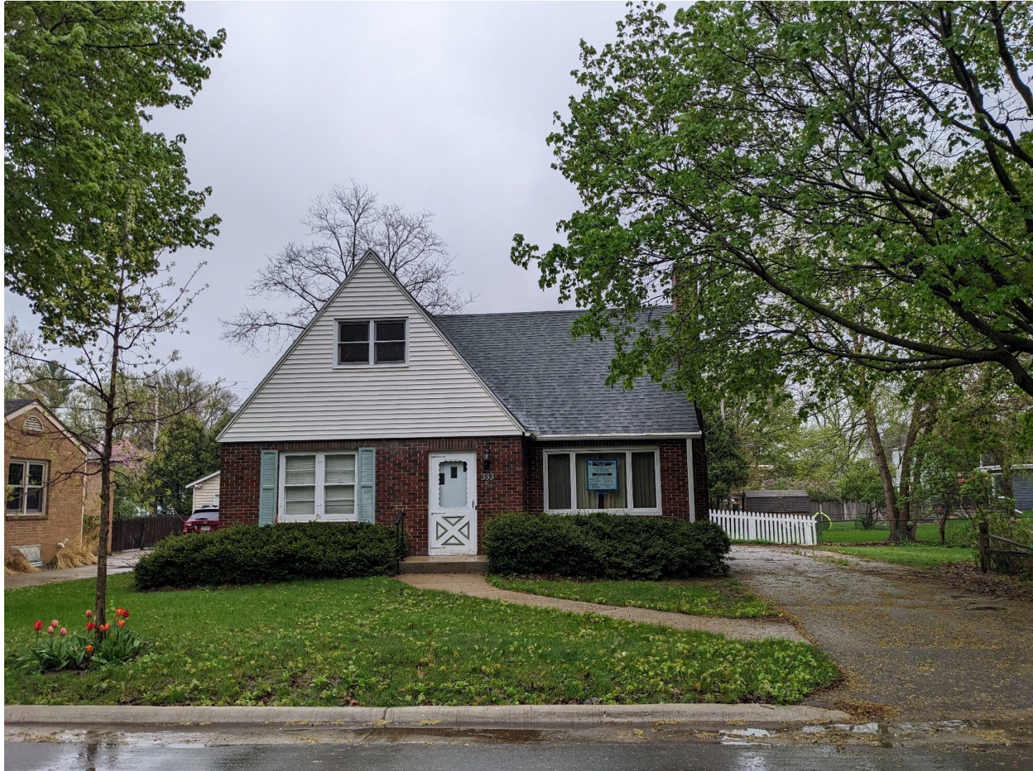
Front West Elevation – View from Sunset Ct
