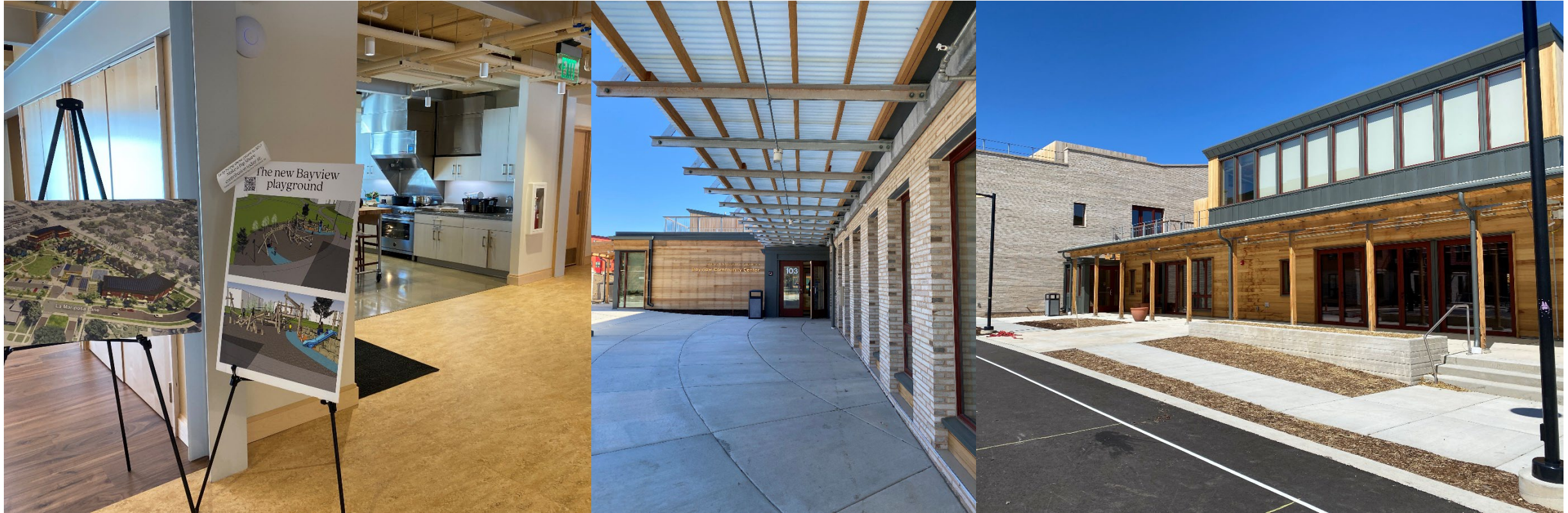
Bayview Community Center
