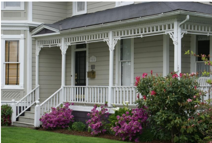
Pre 1900: Typical chamfered columns, simple balustrade and newel posts.
