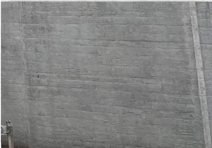
BOARD FORMED CONCRETE
