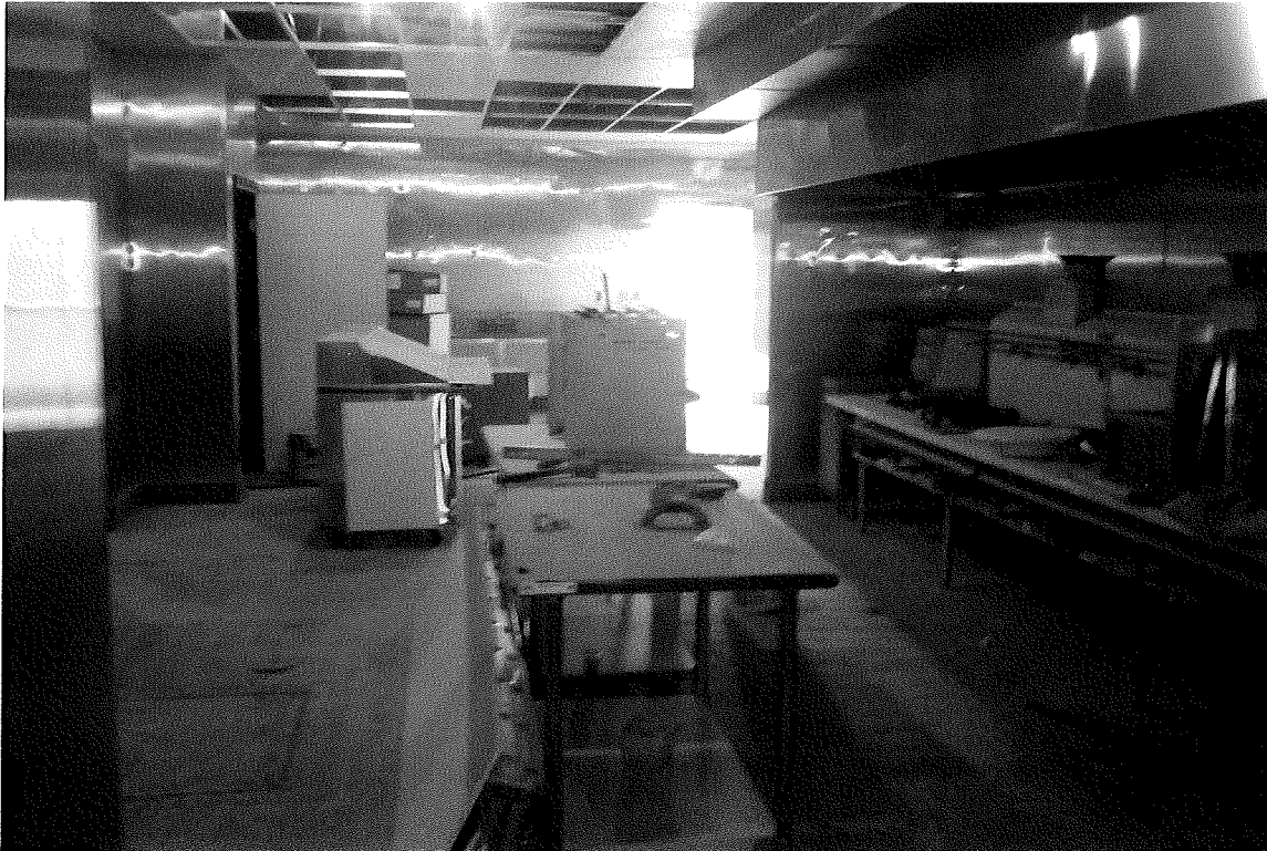
1/2 of kitchen, under construction
