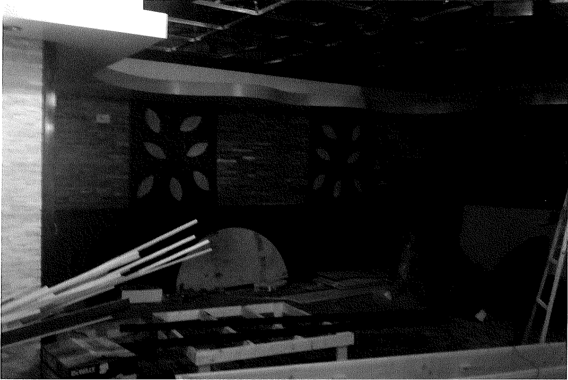
part of dining area under construction
