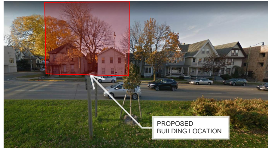
VIEW ALONG E. WASH AVE
