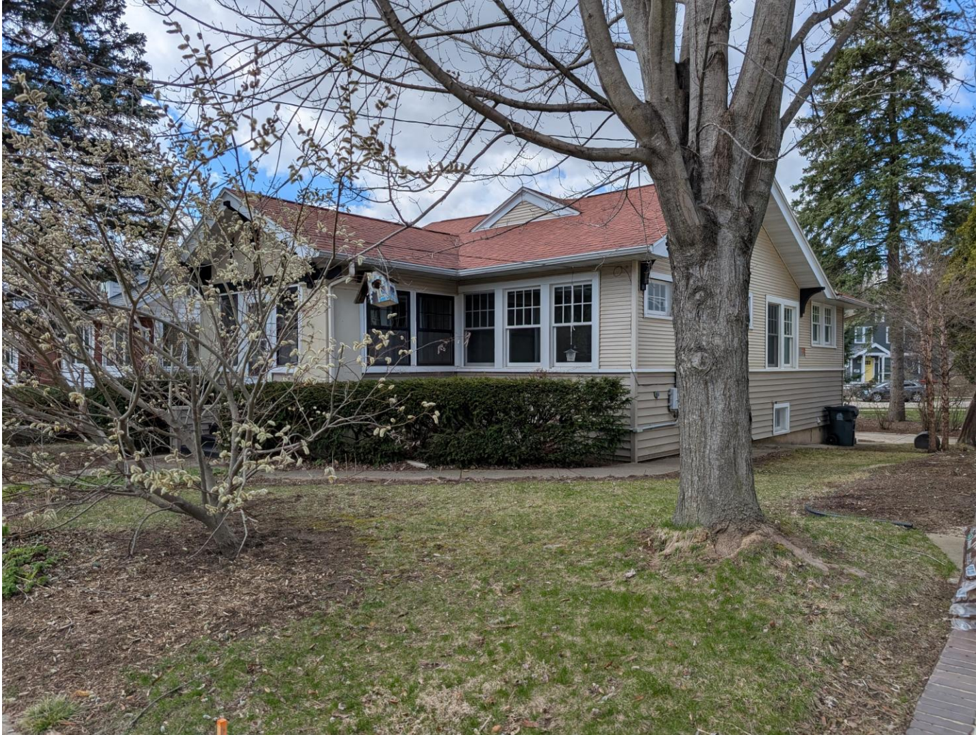
Front and Side of House, Looking Towards Commonwealth Ave
