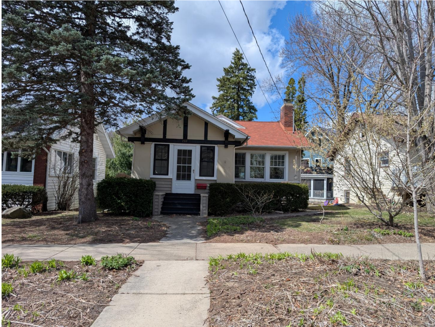
South Front Elevation, view from Keyes Avenue
