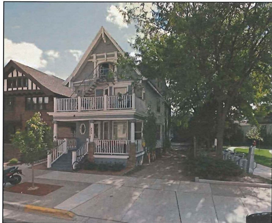
EXISTING BUILDING AND PARK ON GILMAN
