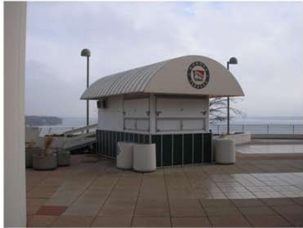
Existing concession kiosk (to be removed)
