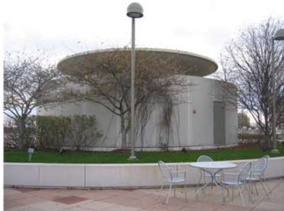
Existing conditions (Fall, looking South)
