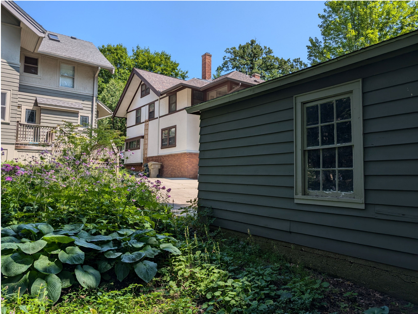
West Side Elevation, Looking North Towards Van Hise
