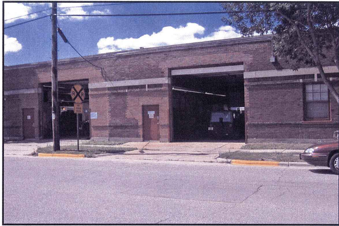
EXISTING BUILDING - LOOKING WEST
