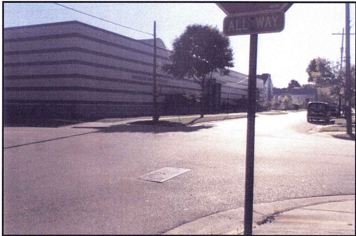
PATERSON STREET - LOOKING SOUTHEAST
