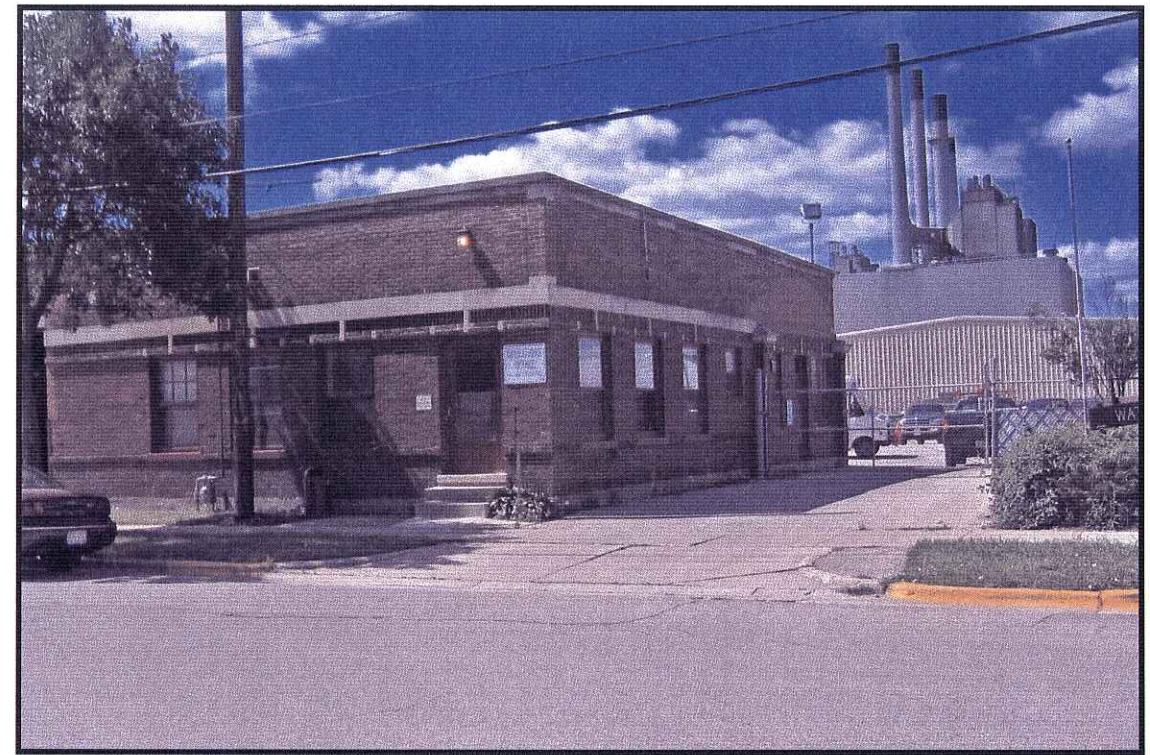
EXISTING BUILDING - LOOKING WEST
