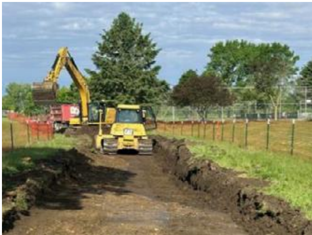
Pictured above: (left) topsoil removal on future bike path, (right) on-site signage. Photos provided by CCI.
