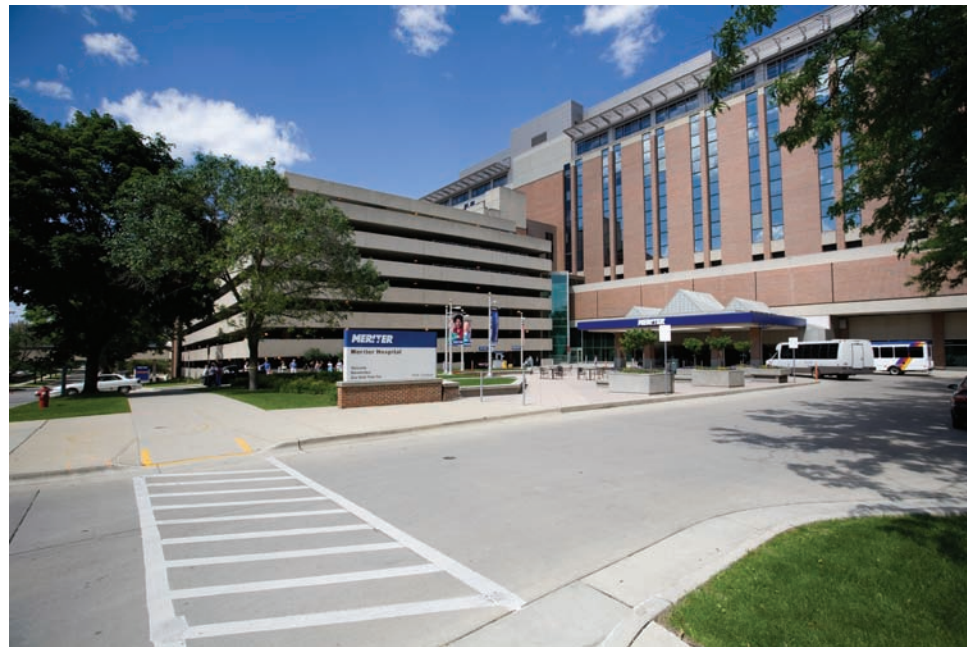
existing site condition
