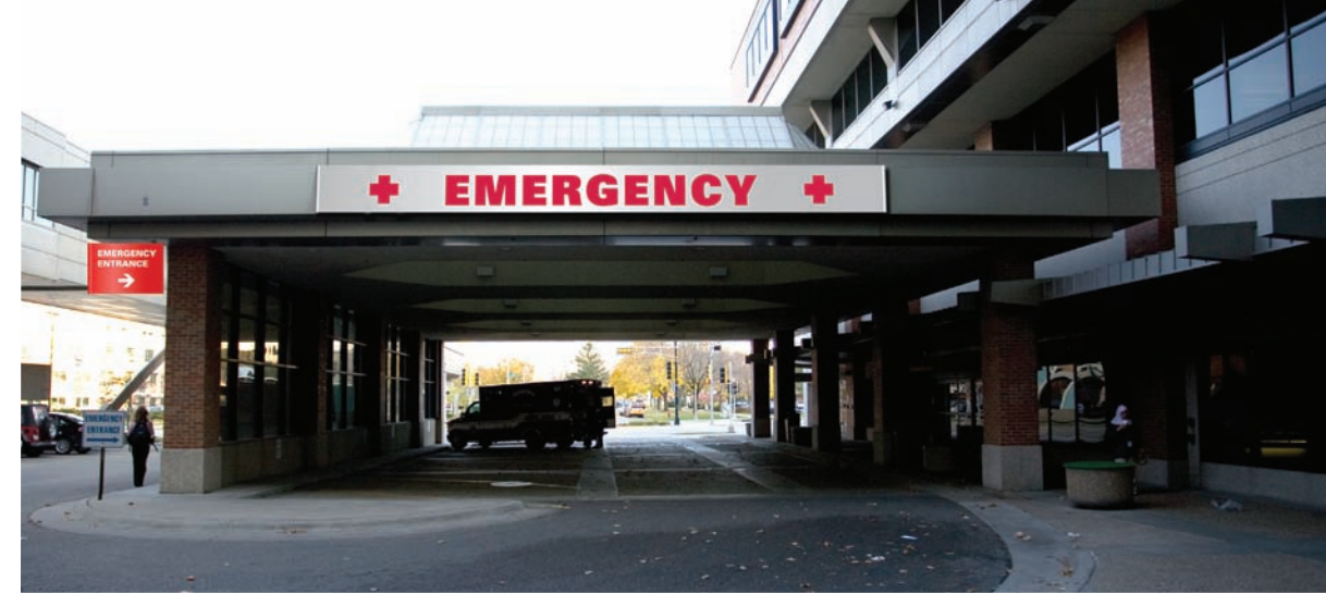
2 Emergency Canopy West Side Internally Illuminated Aluminum Sign Cabinet 30' L x 2'8" H x 0'-4" D overall 84 sq ft signable area
