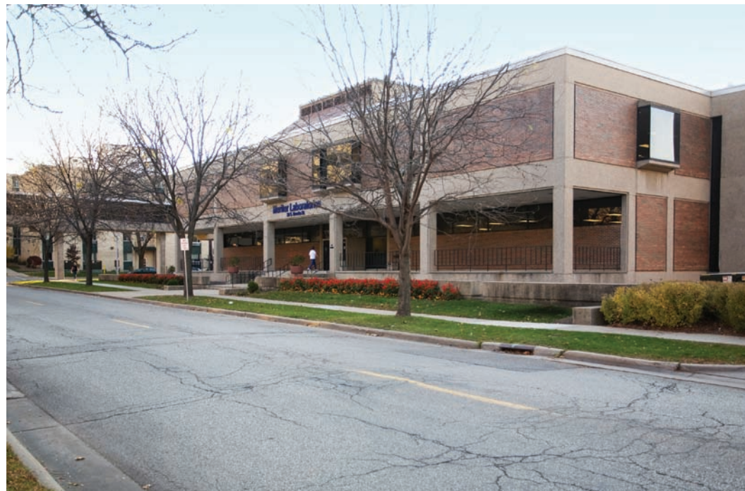
existing site condition
