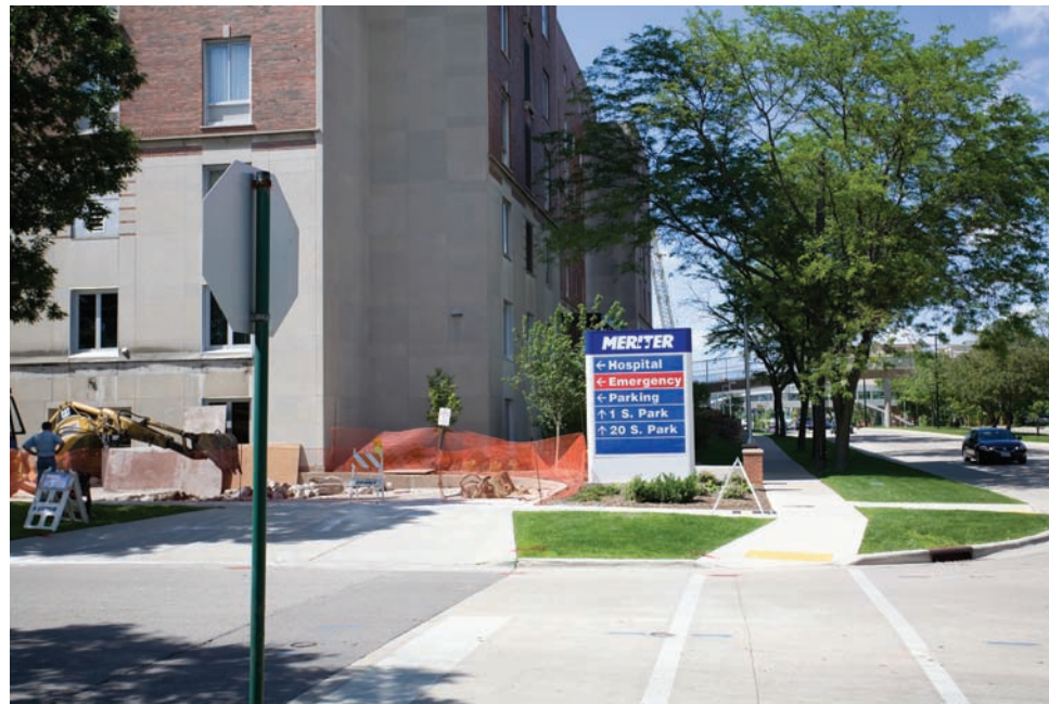
existing site condition
