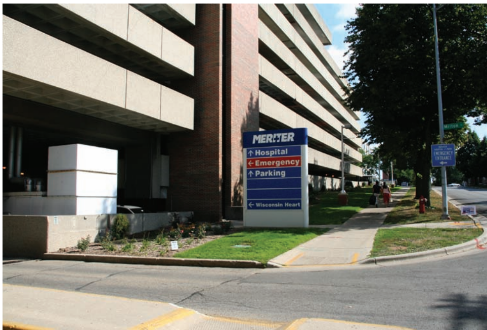
existing site condition
