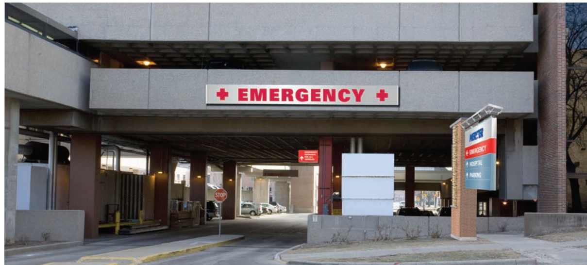
3 Emergency Entrance on Mound Street Internally Illuminated Aluminum Sign Cabinet 25'10" L x 2'8" H x 0'-4" D overall 84 sq ft signable area
