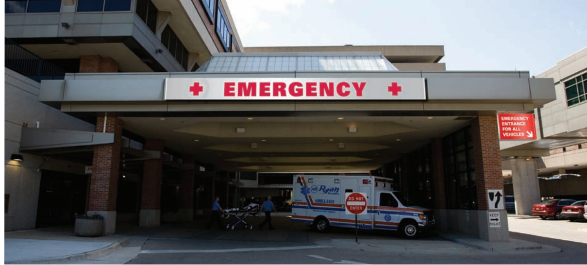
1 Emergency Canopy Facing Park Street Internally Illuminated Aluminum Sign Cabinet 30' L x 2'8" H x 0'-4" D overall 84 sq ft signable area
