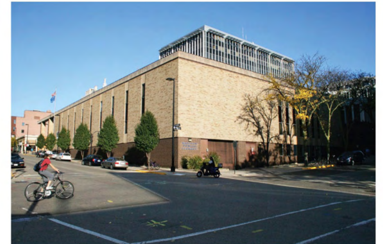
VIEW FROM MIFFLIN STREET AND HENRY STREET
