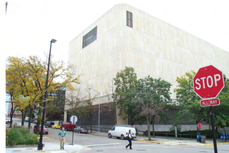
BUILDING ACROSS HENRY STREET
