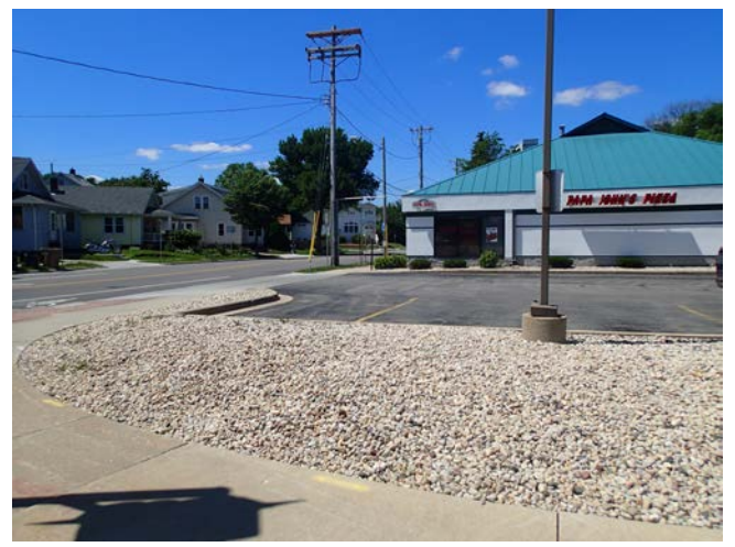
Focus Area Two Existing Conditions
