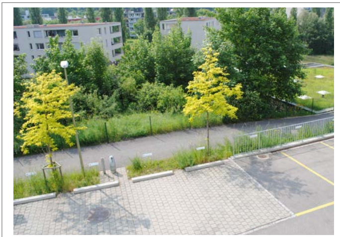
Permeable parking strip drains to grassy swale to protect stream quality, Futuro Office Park in Liestal Switzerland Photo Laura Tam
