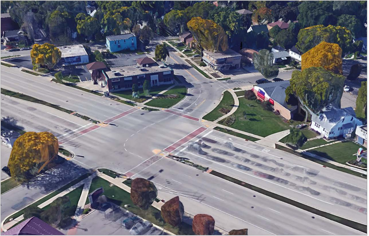
Figure 1a. Focus Area One Existing Conditions
