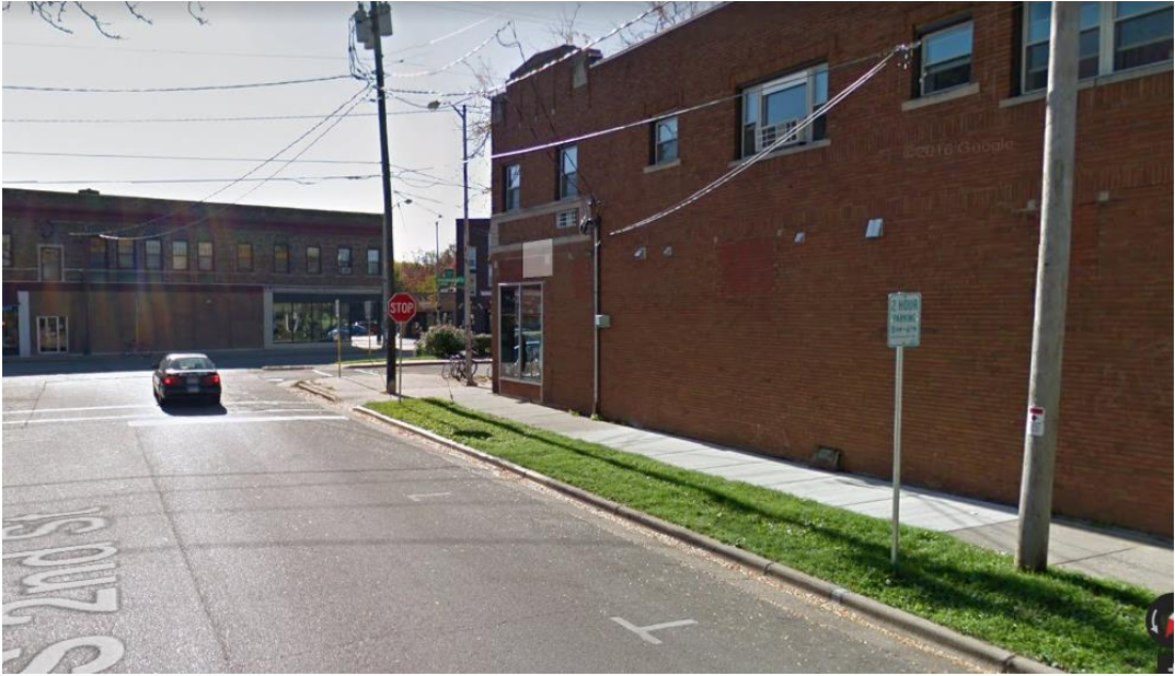
Location #7: Alchemy (1980 Atwood Ave) Hinged Sign on existing pole on 2 nd Street with arrow pointing towards intersection.
