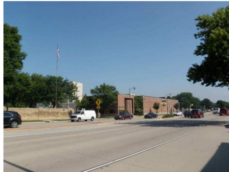
VIEW FROM EAST WASHINGTON LOOKING NORTHEAST
