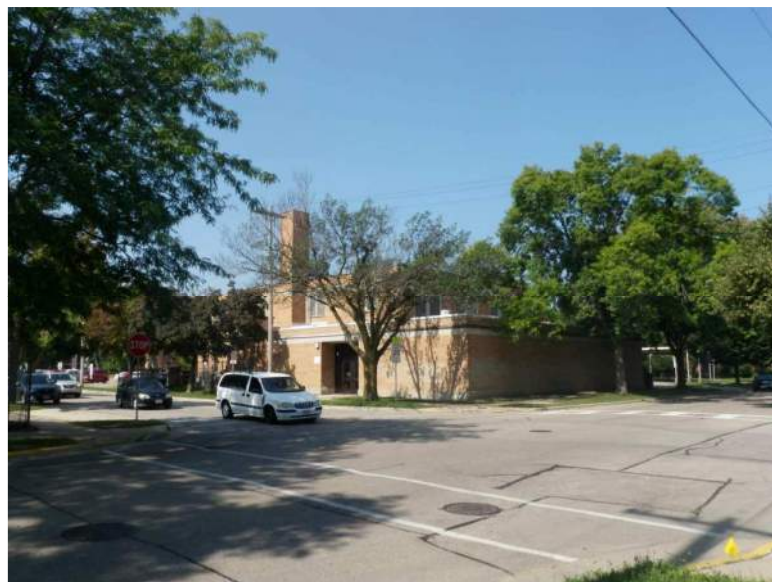
VIEW FROM MIFFLIN AND INGERSOLL LOOKING WEST
