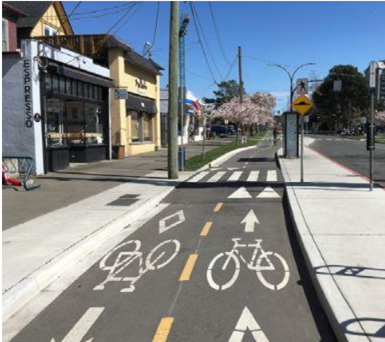
Figure B.4-7 Vancouver, BC – Two-way cycletrack at street level with raised pedestrian crossing
