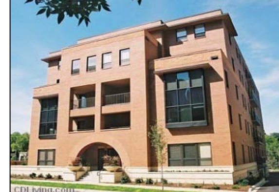
Apartment Building 22 E Dayton 3.0 FAR
