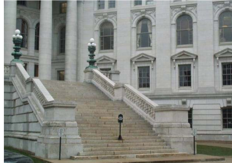
State Capitol Stair is Approximately 17'-7"
