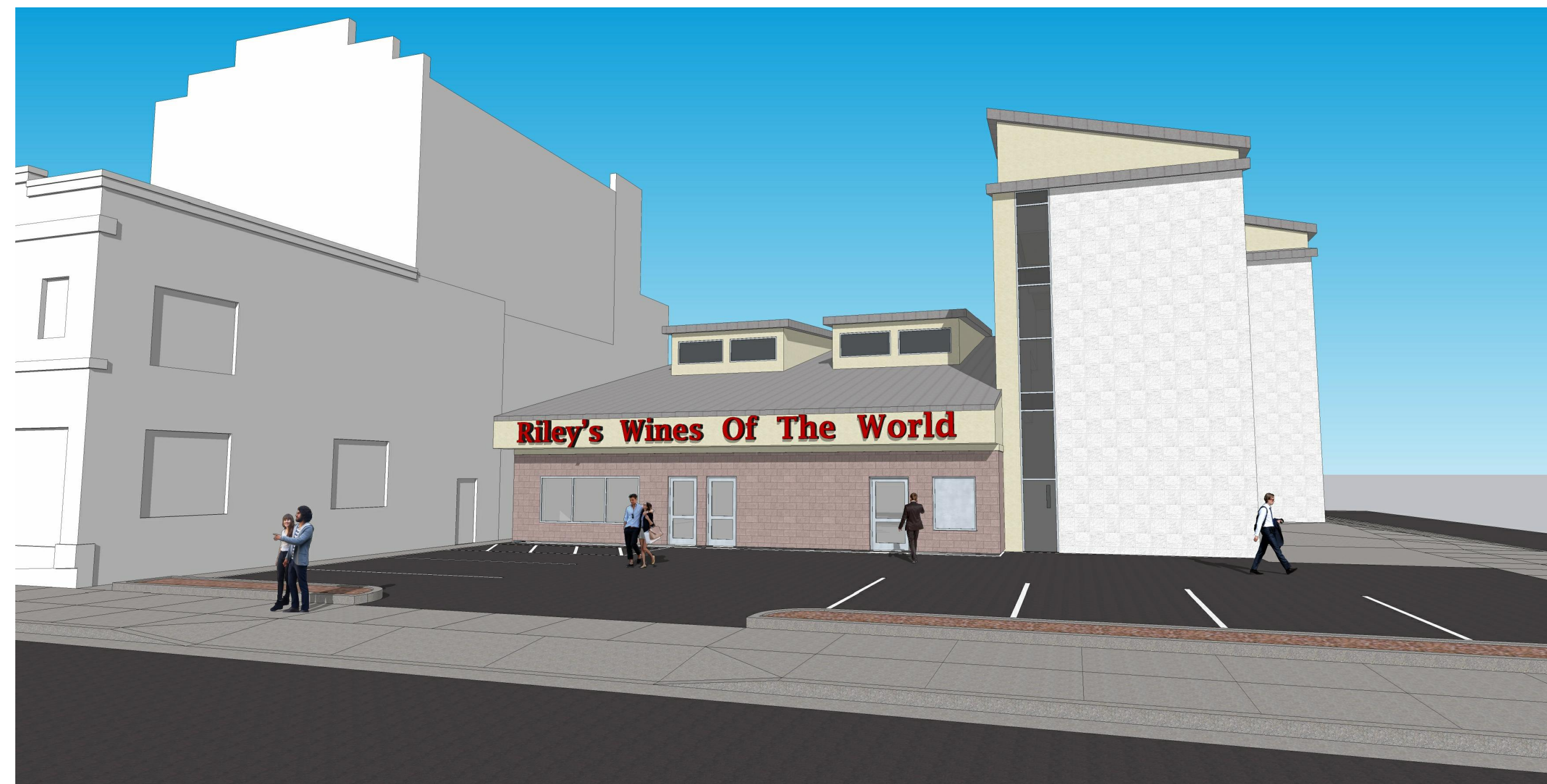
1 EXISTING BUILDING FROM GORHAM STREET SCALE: NTS
