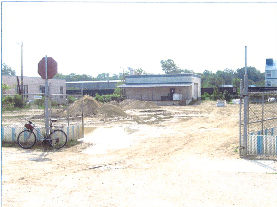
VIEW OF ENTRY FACING SOUTH
