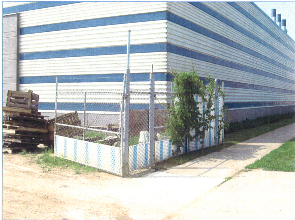
VIEW OF ENTRY FACING WEST
