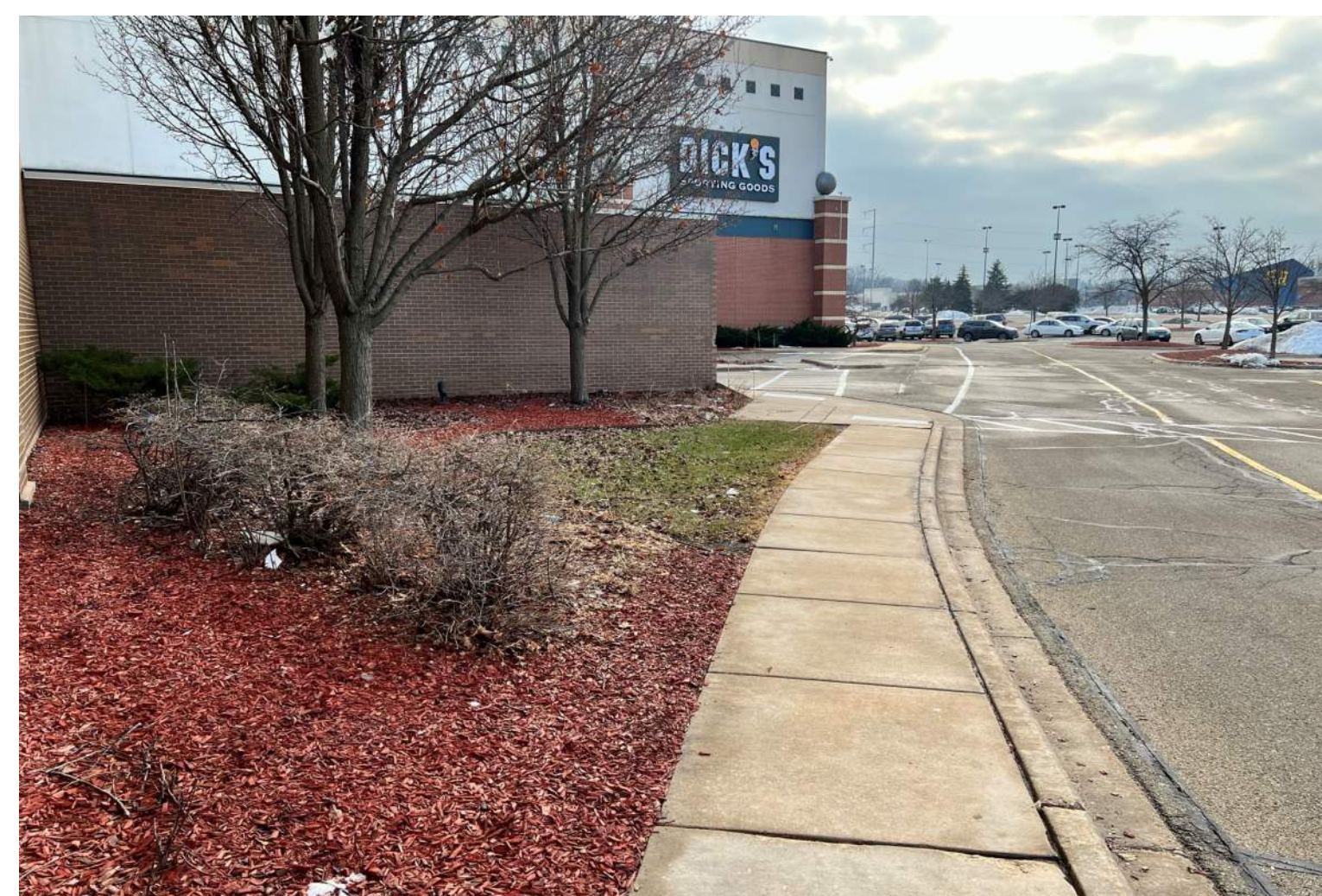
DICK'S SPORTING GOODS NORTH EXTERIOR WALL
