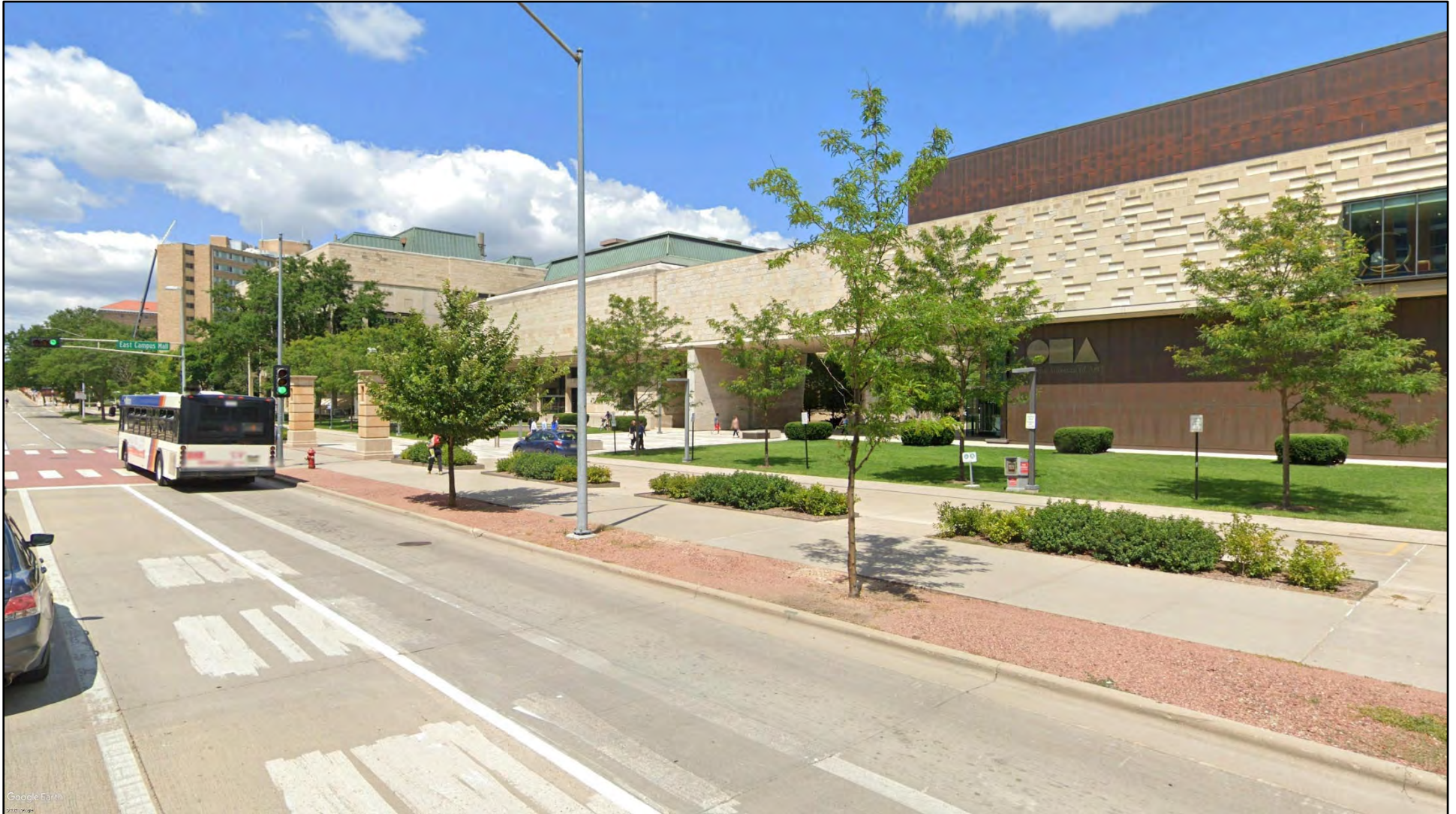
Figure 18. University Avenue at Campus Mall, View Northwest – Existing Adjacent to Bascom Hill Historic District, 2011 Chazen Museum of Art Expansion (Noncontributing) in Background at Right
