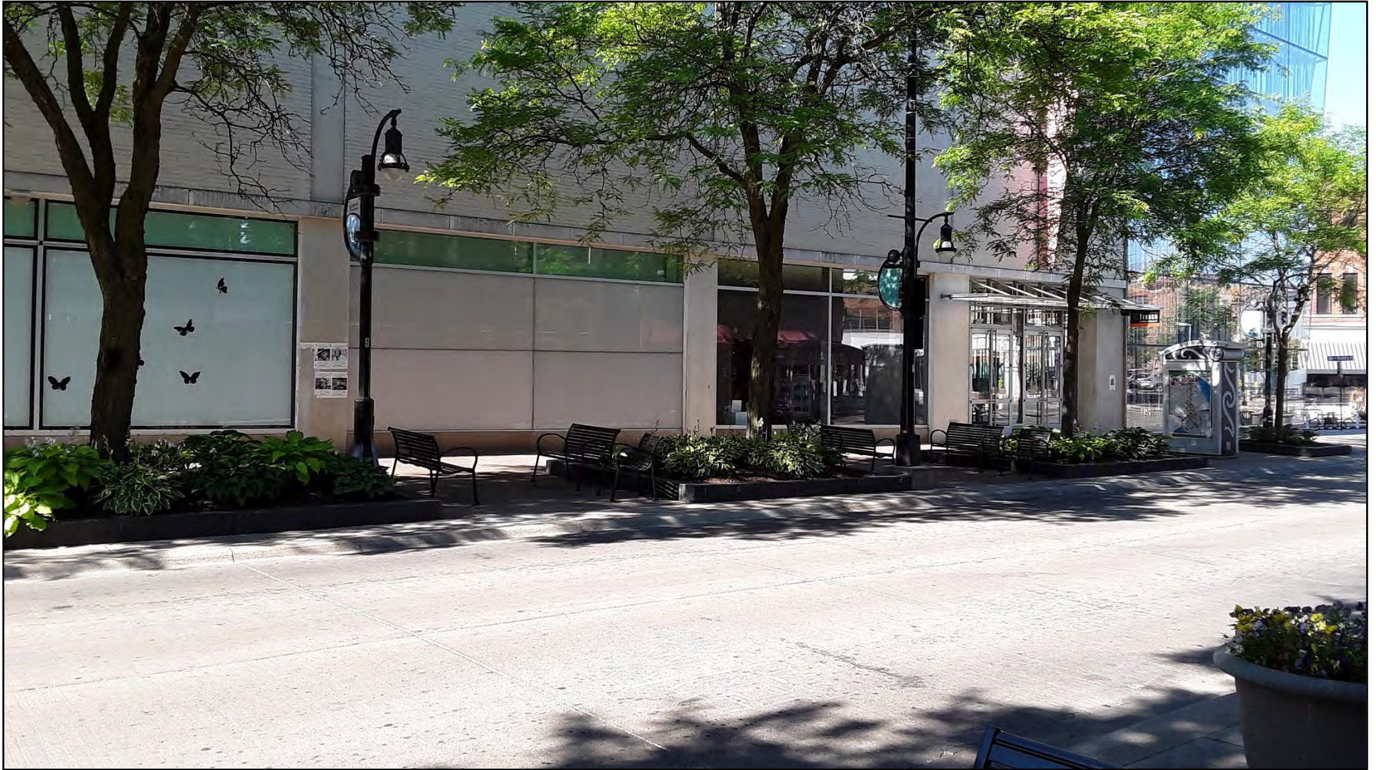
Figure 27. State Street at Johnson Street, View Southwest – Existing Within State Street Historic District, Madison Museum of Contemporary Art (Noncontributing) in Background
