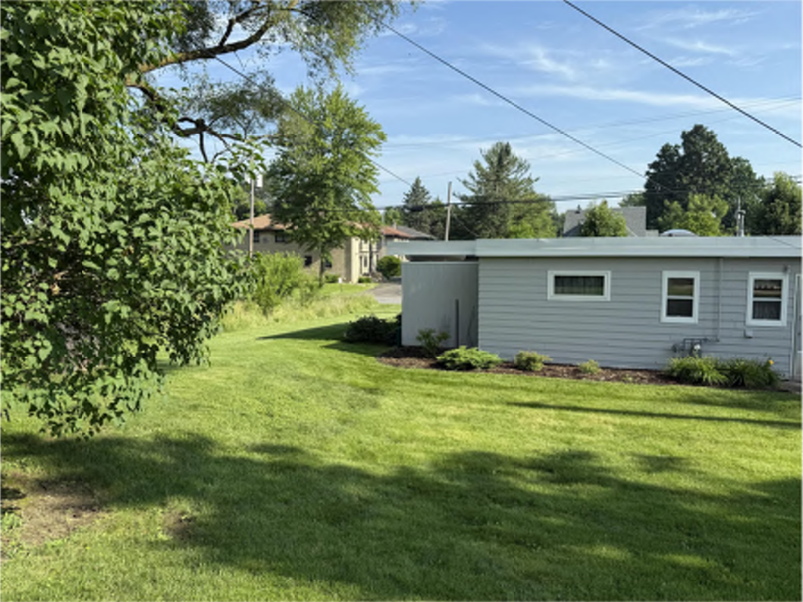
LOOKING NORTH RESIDENCES ARE OCCUPIED AND COULD BE ENTERED
