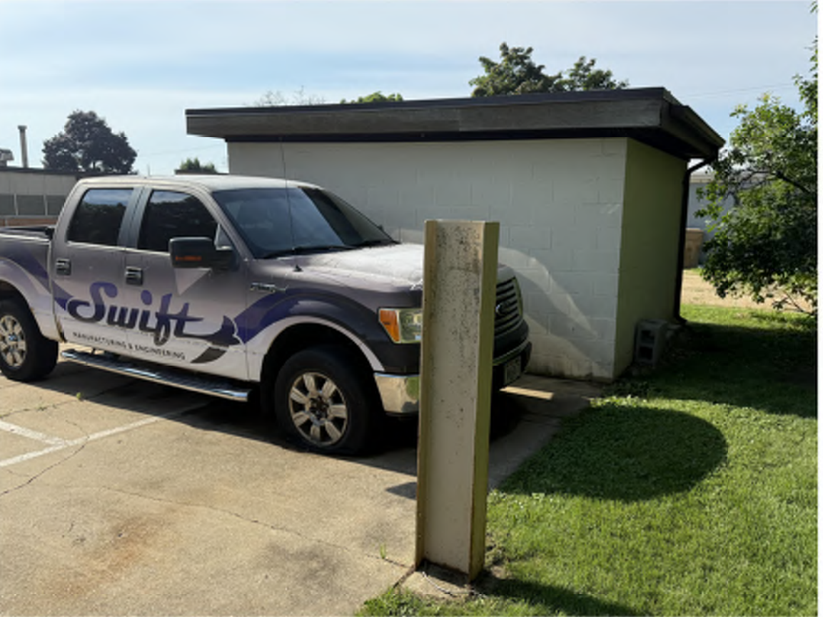
ABANDONED VEHICLE AND STORAGE BUILDING BUSINESS IN USE AND ACCESS TO THE INTERIOR WAS NOT OBTAINED
