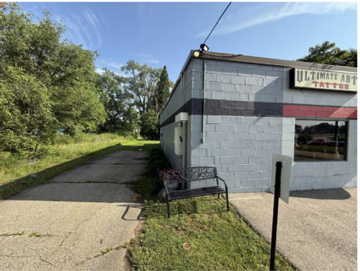
WEST SIDE OF BUILDING
