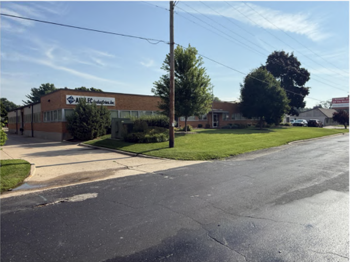
VIEW NORTHWEST ALONG COMMERCIAL AVENUE
