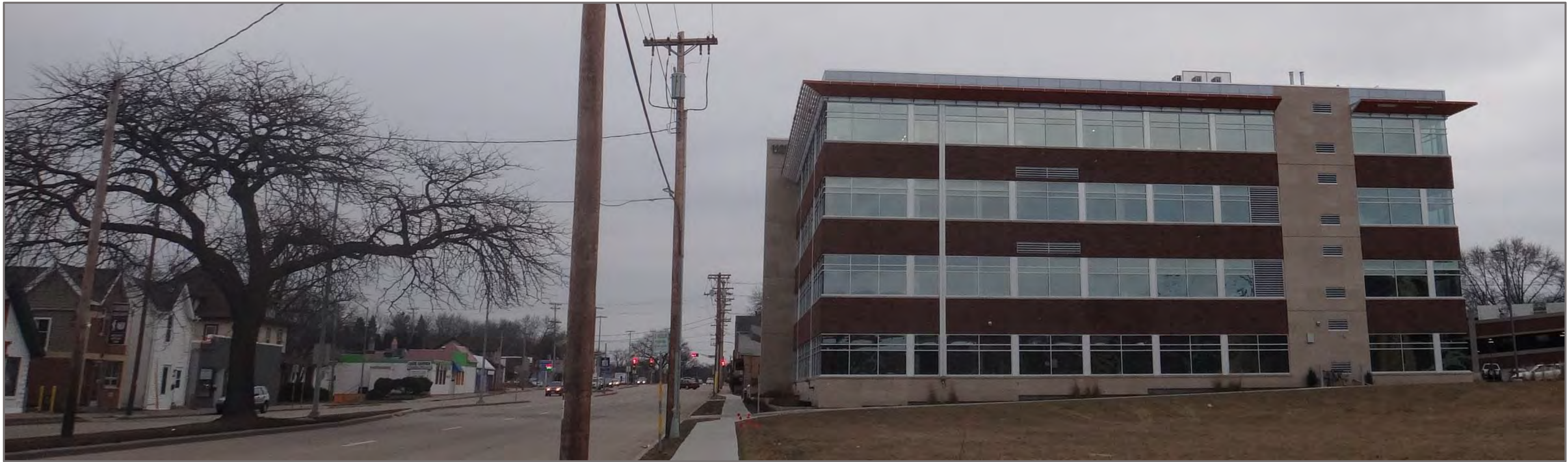
Wingra Clinic –View Looking South from Park St
