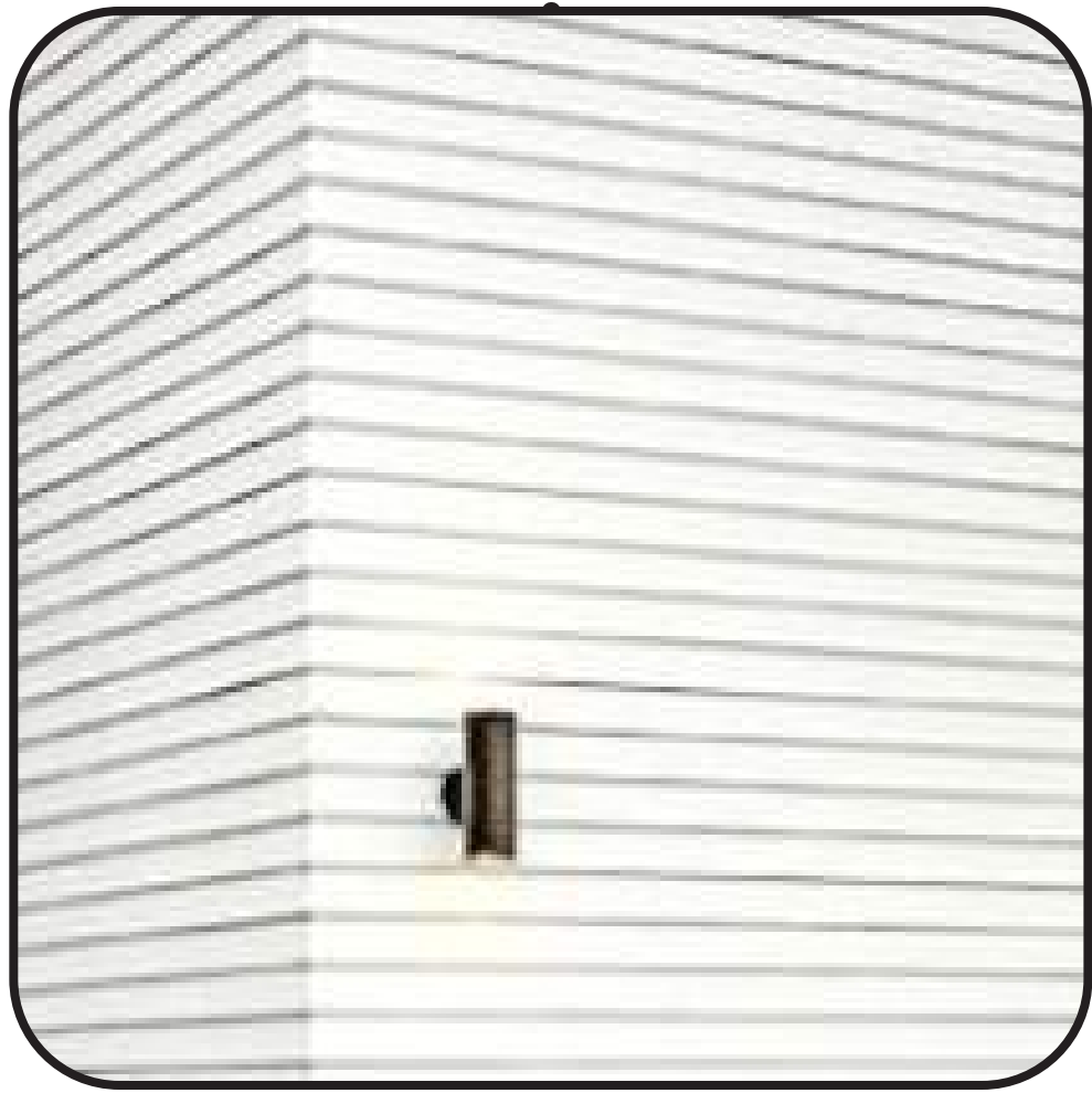
FIBER-CEMENT - LAP SIDING
