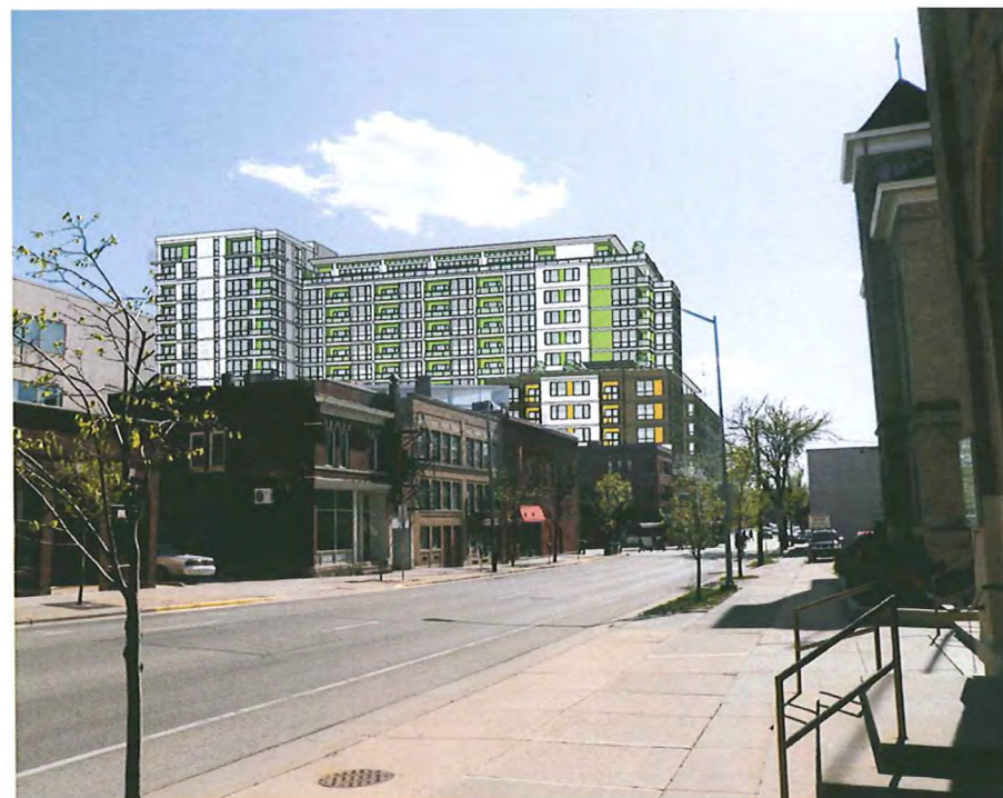
View From Johnson Street
