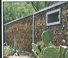
Rock Wall Fencing
