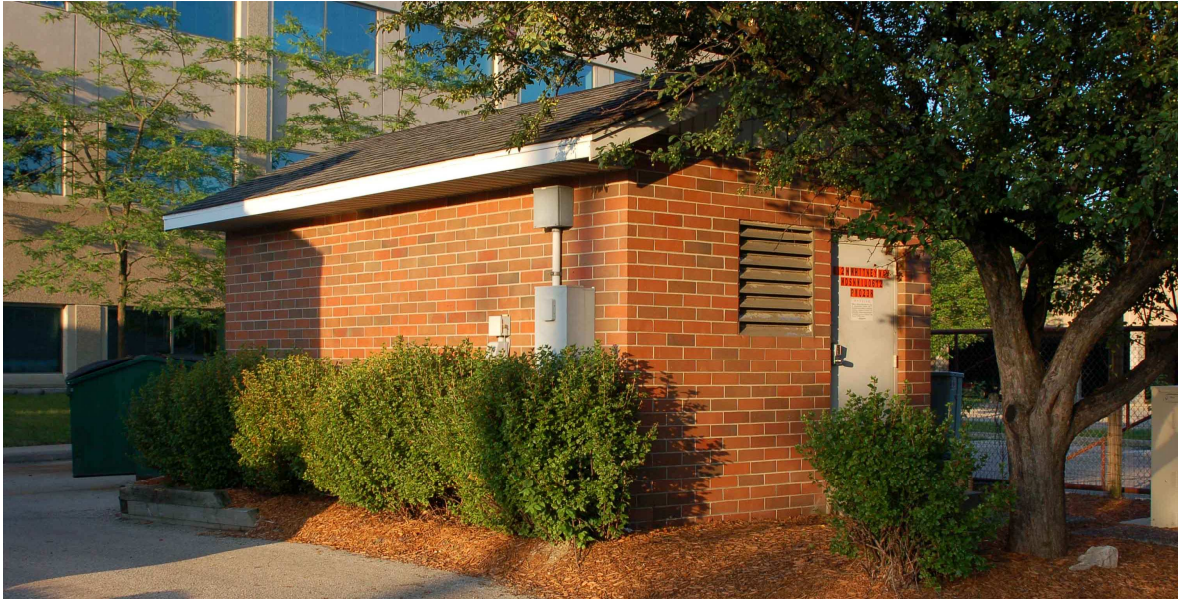
Easement, "AT+T Utility Shed"
