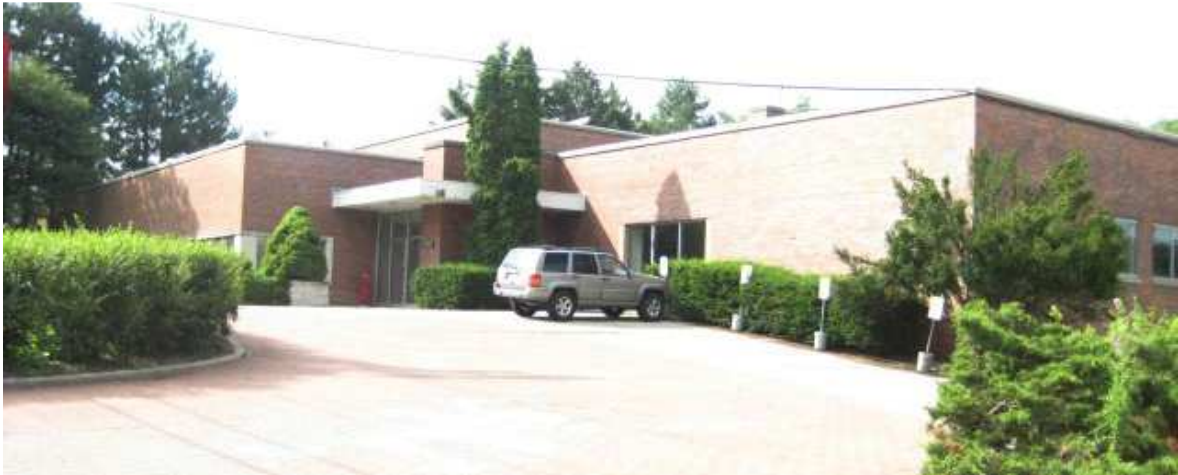
5105 University Avenue, "Building 2"
