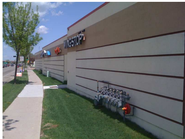
Figure 3d: Back of retail building facing Gammon Road.
