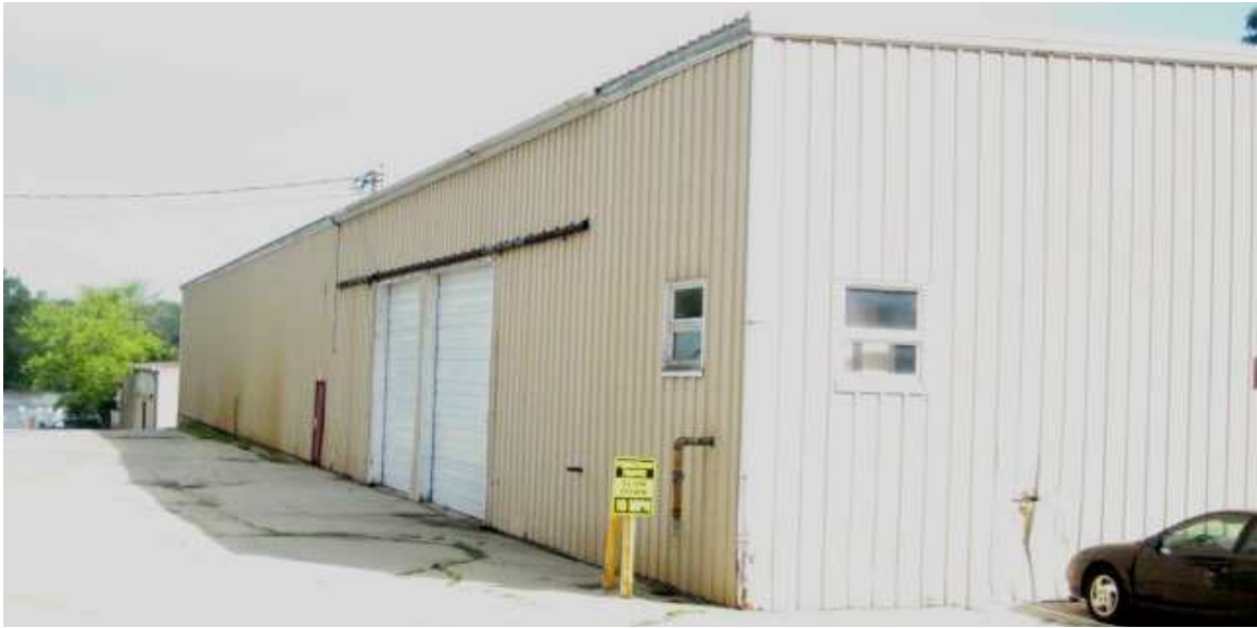
5115 University Avenue, "Upper Warehouse"
