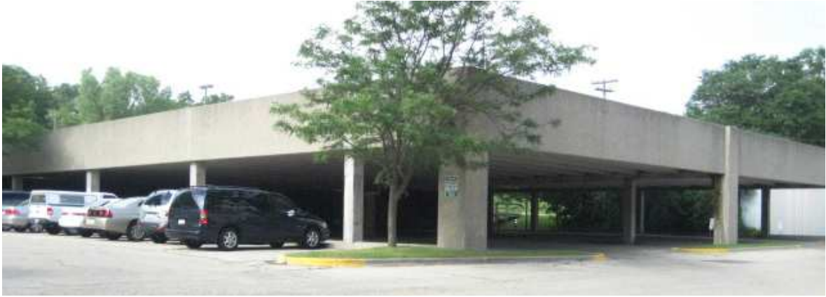
610 N. Whitney Way, "PSC Parking Ramp"
