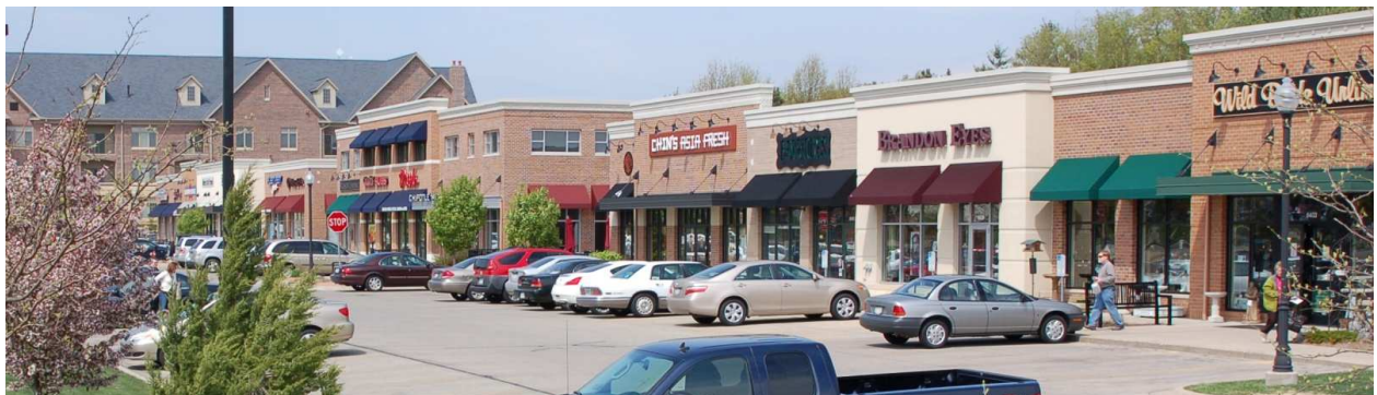
Figure 3e: Fronts of retail stores facing the street: people, window displays and activity create a pleasant face to the street.
