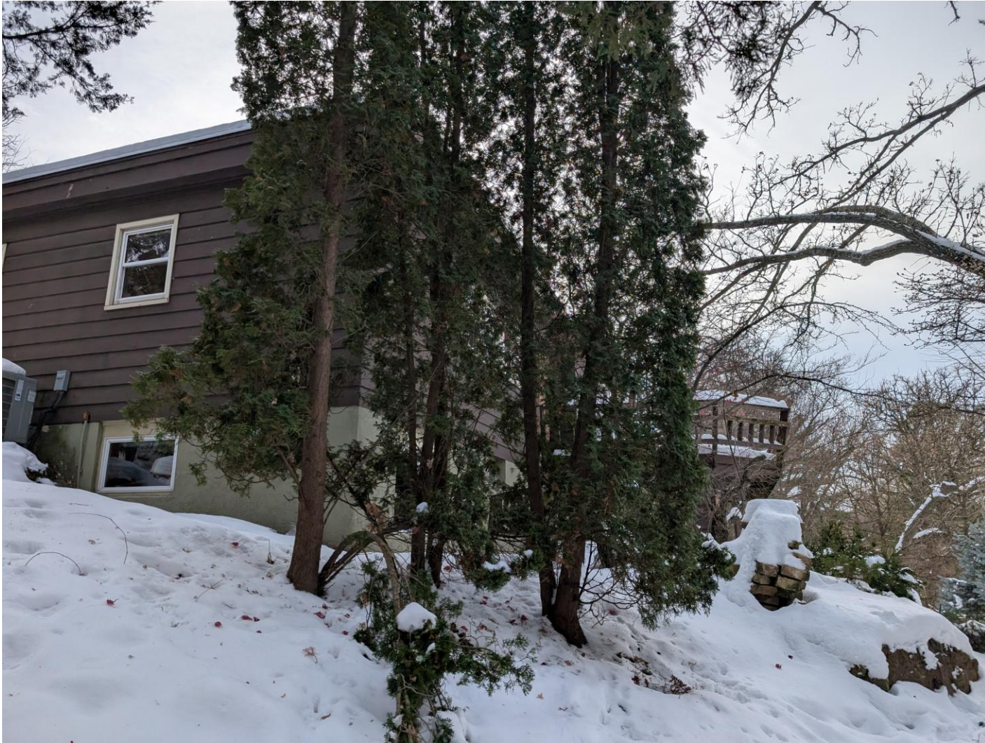
East Side and Front North Elevation
