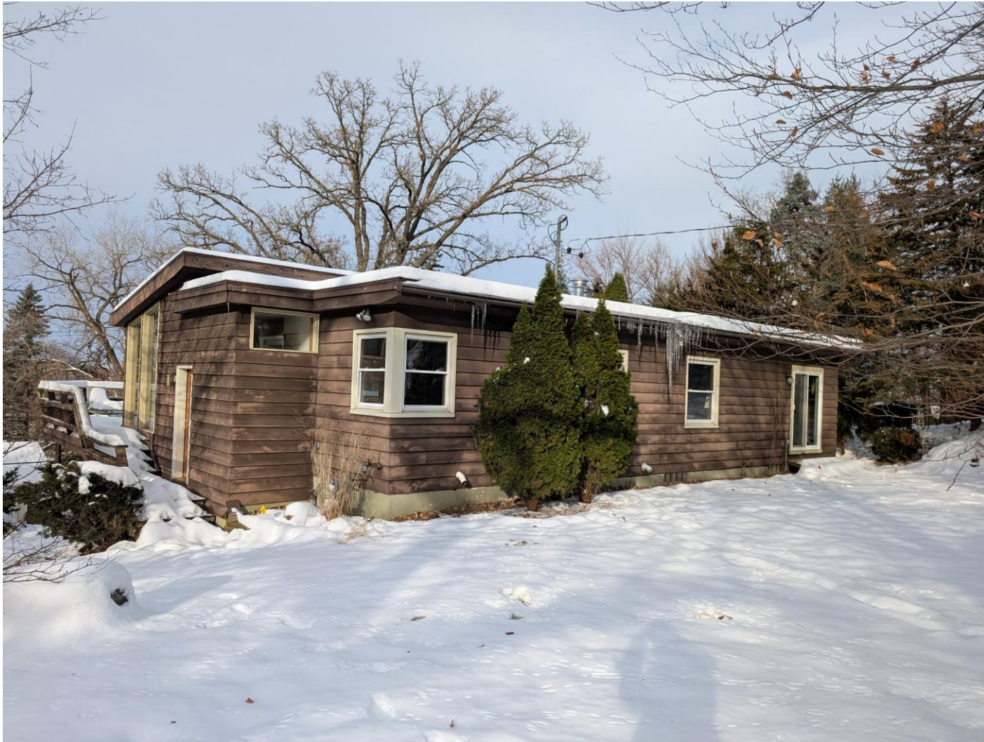
West Side and South Rear Elevation
