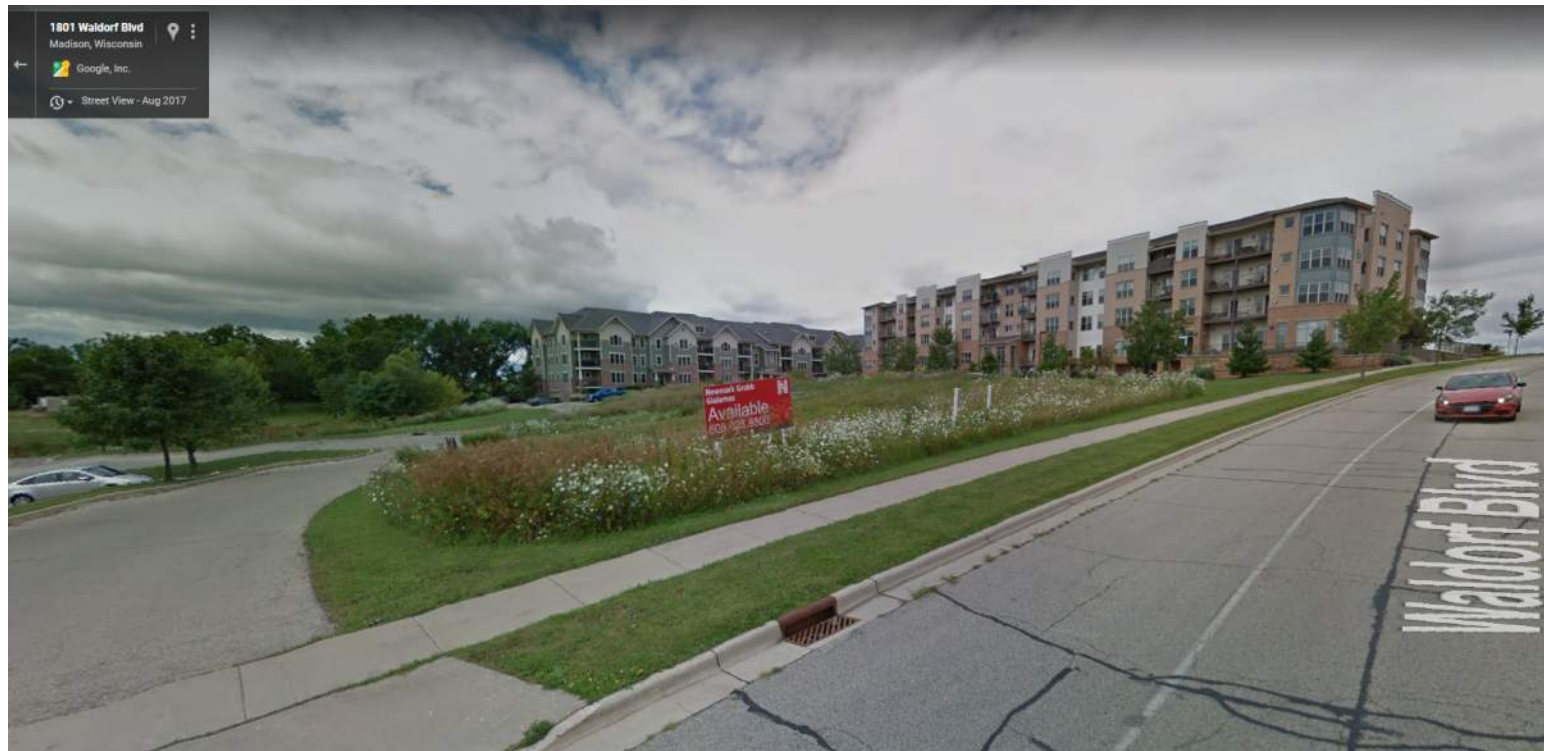
WALDORF BOULEVARD AT PRIVATE ROAD - LOOKING NORTH WEST
