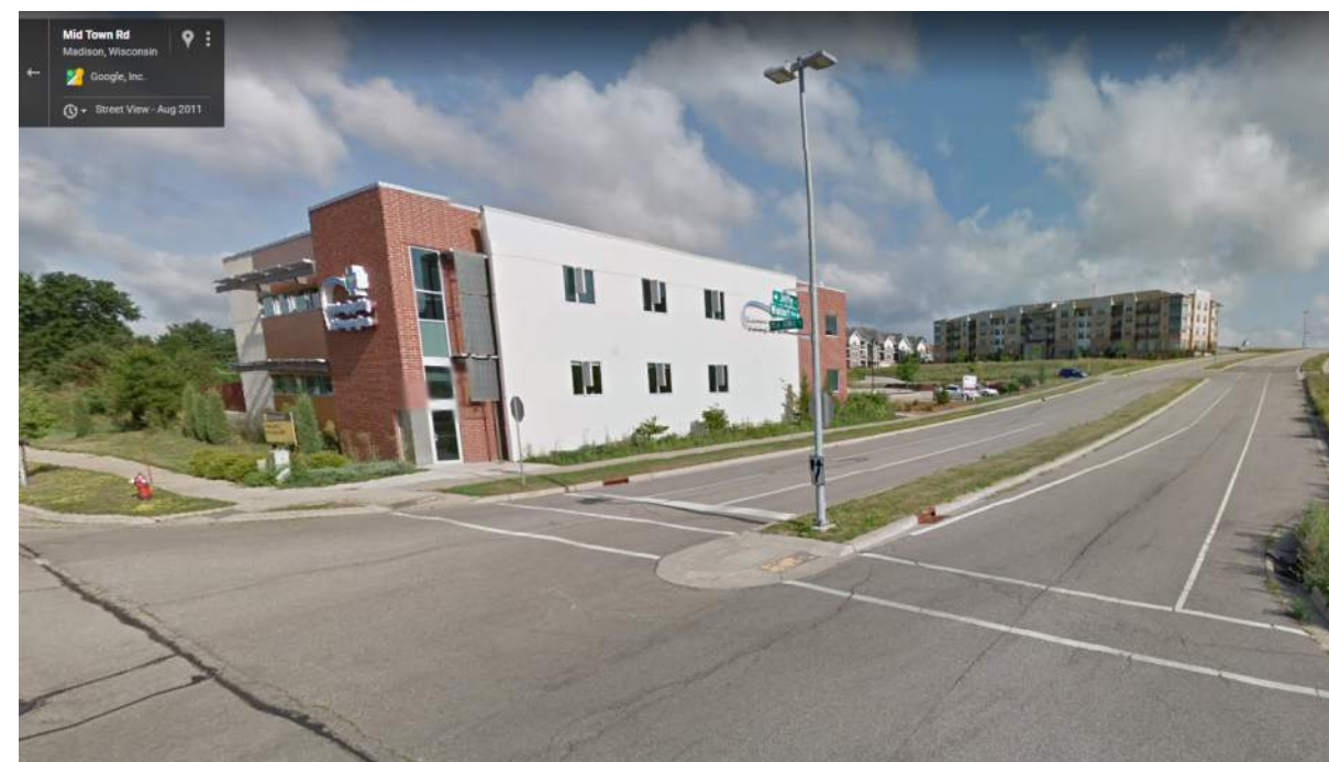
MIDTOWN ROAD AND WALDORF BOULEVARD - LOOKING NORTH EAST
