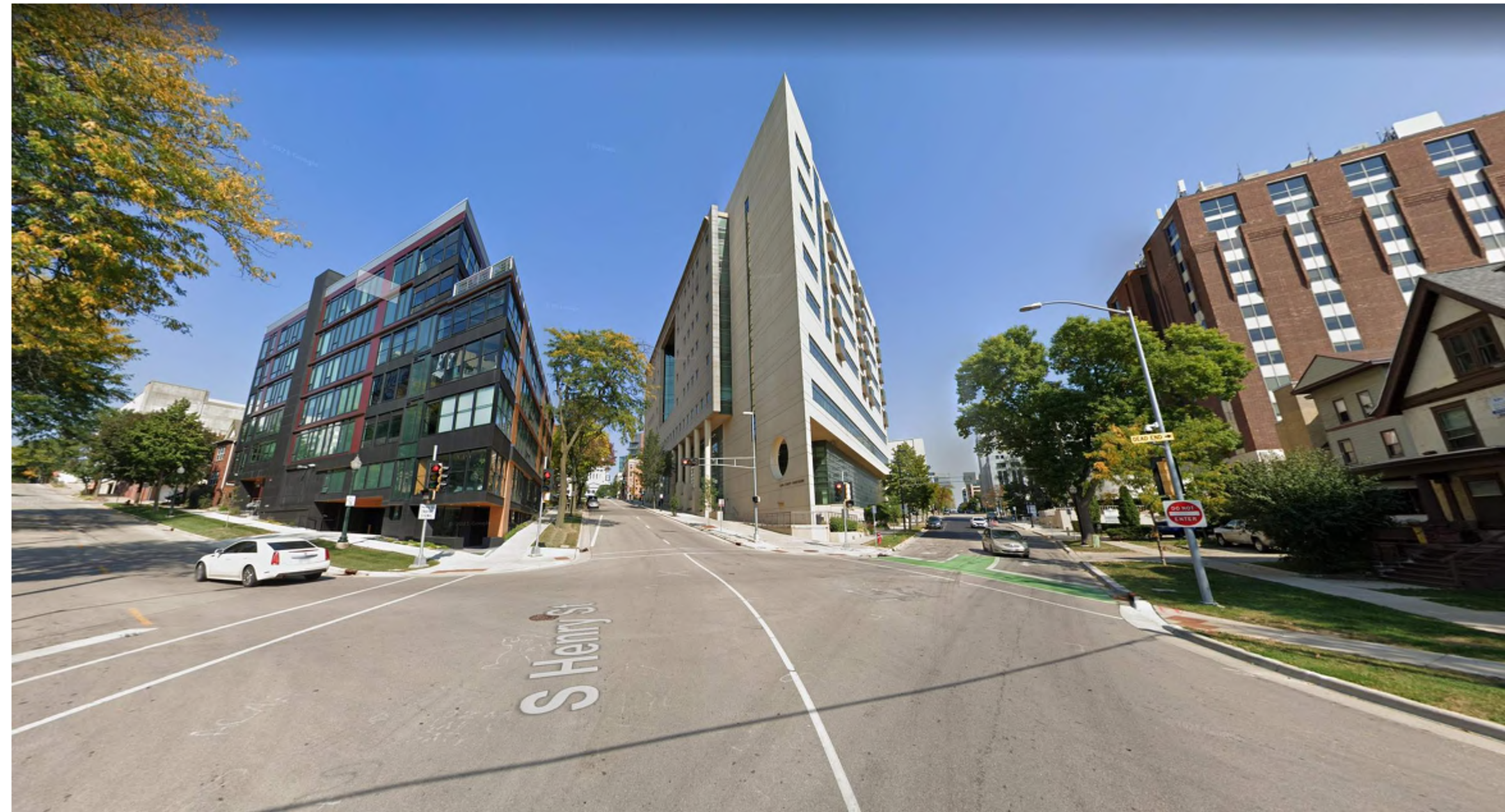
VIEW LOOKING NORTH AT HAMILTON STREET
