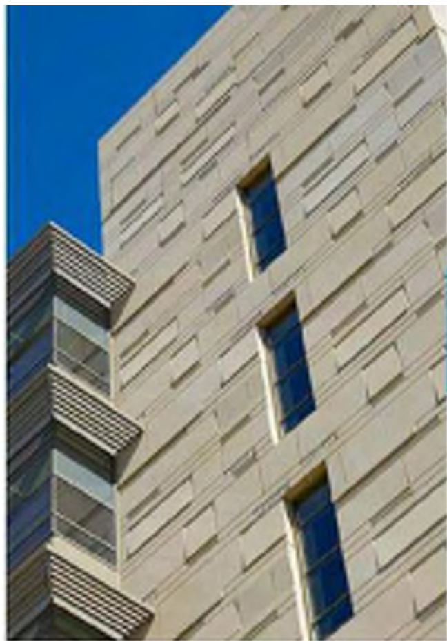
Acid etched concrete wall panel. Color: PEARL WHITE
