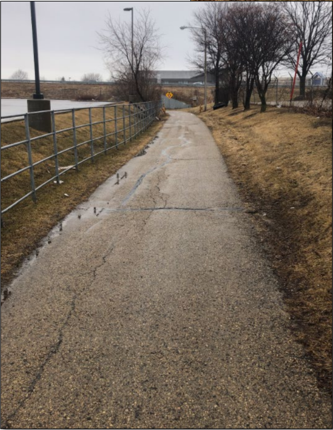
South Side – To Be Replaced
