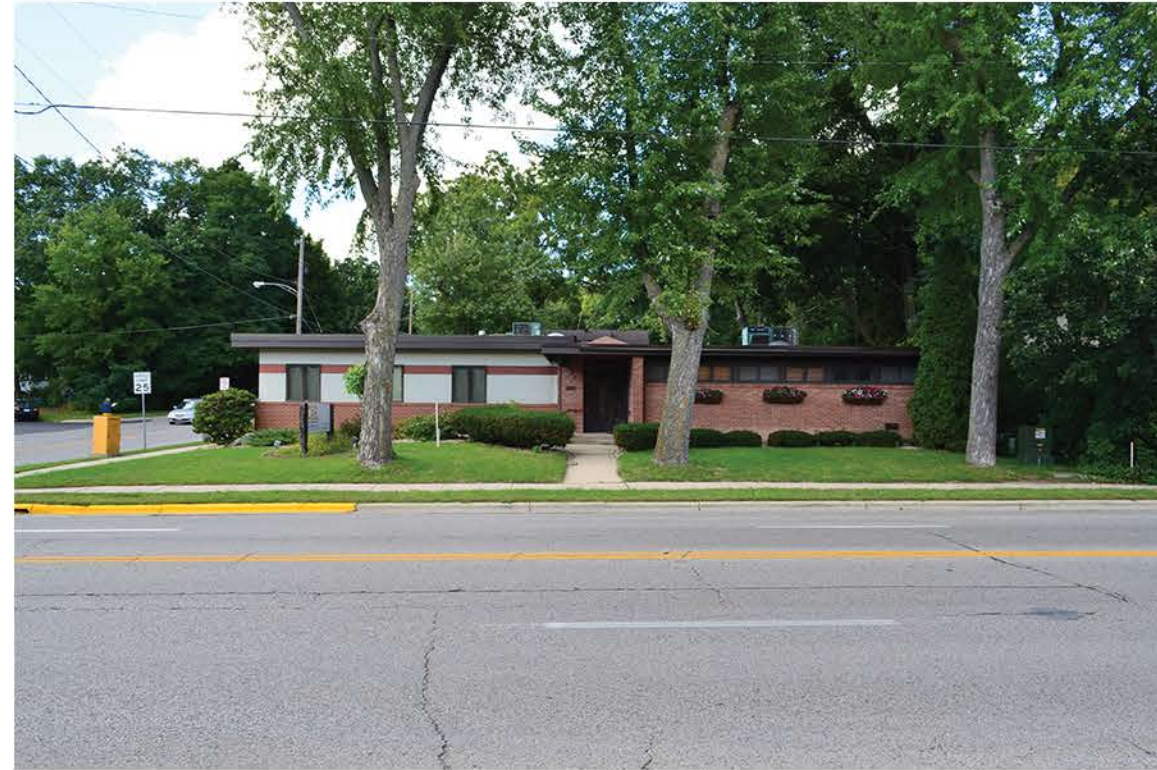
Existing Building along Monroe Street
