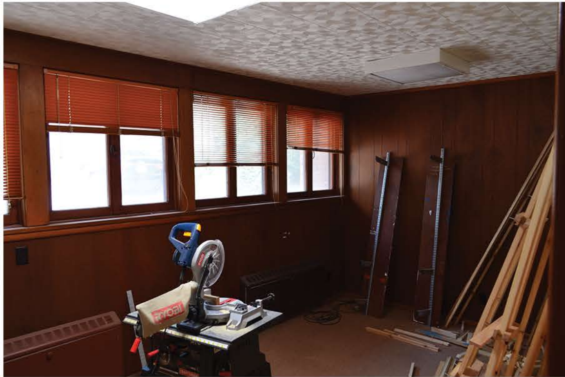
Existing Office Area within original building
