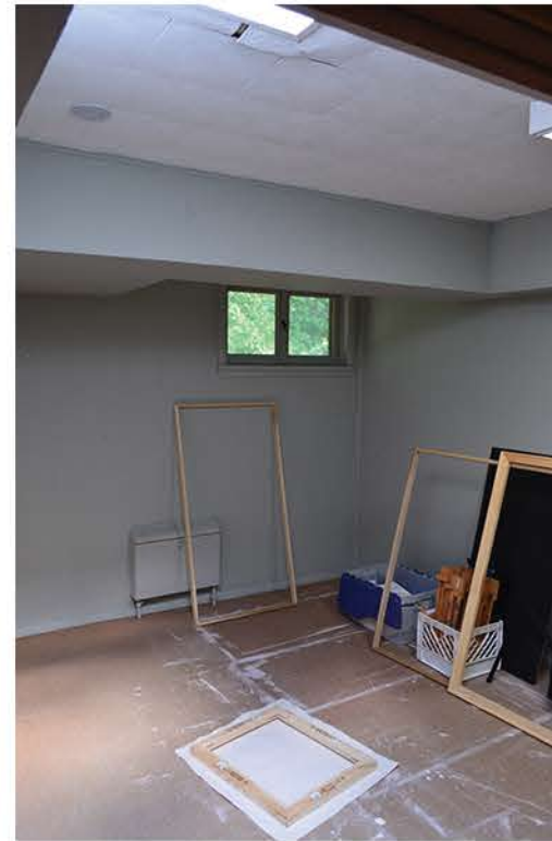
Existing Office Area within original building
