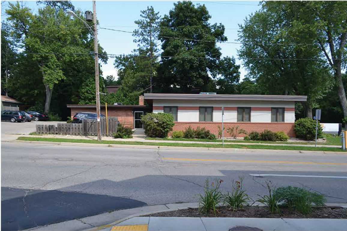
Existing Building along Glenway Street
