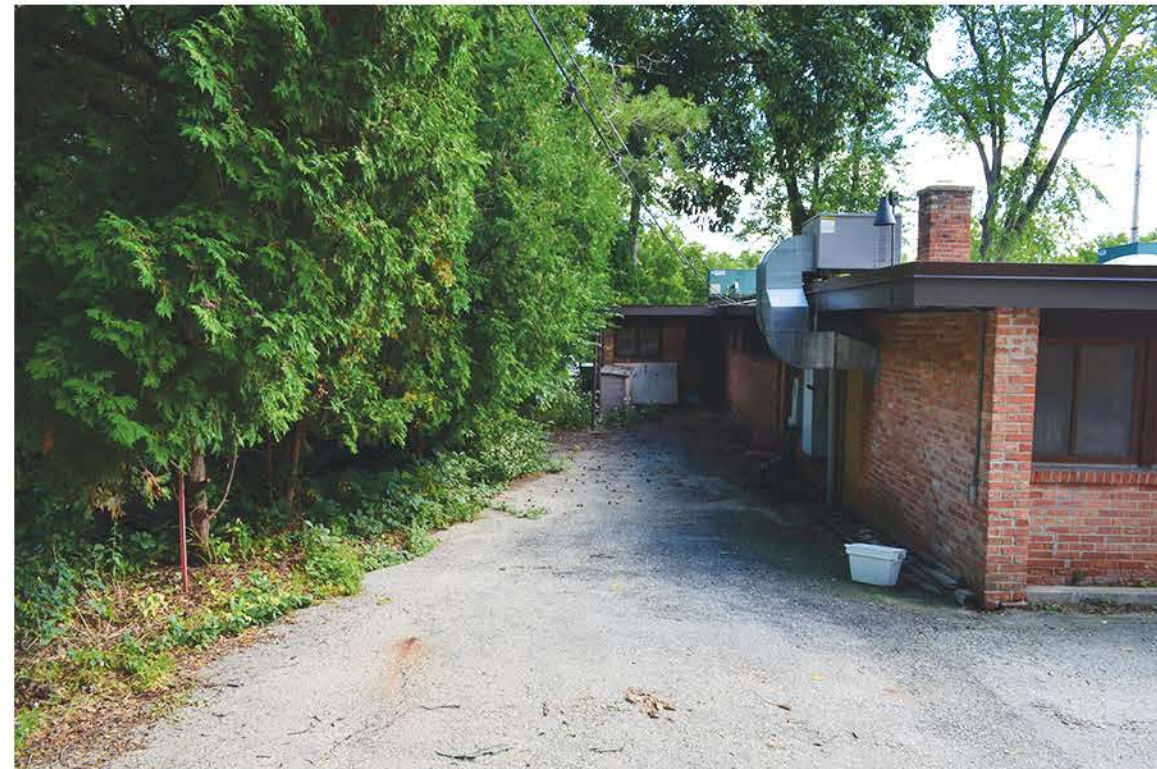
Existing Building adjacent to Arbor House property
