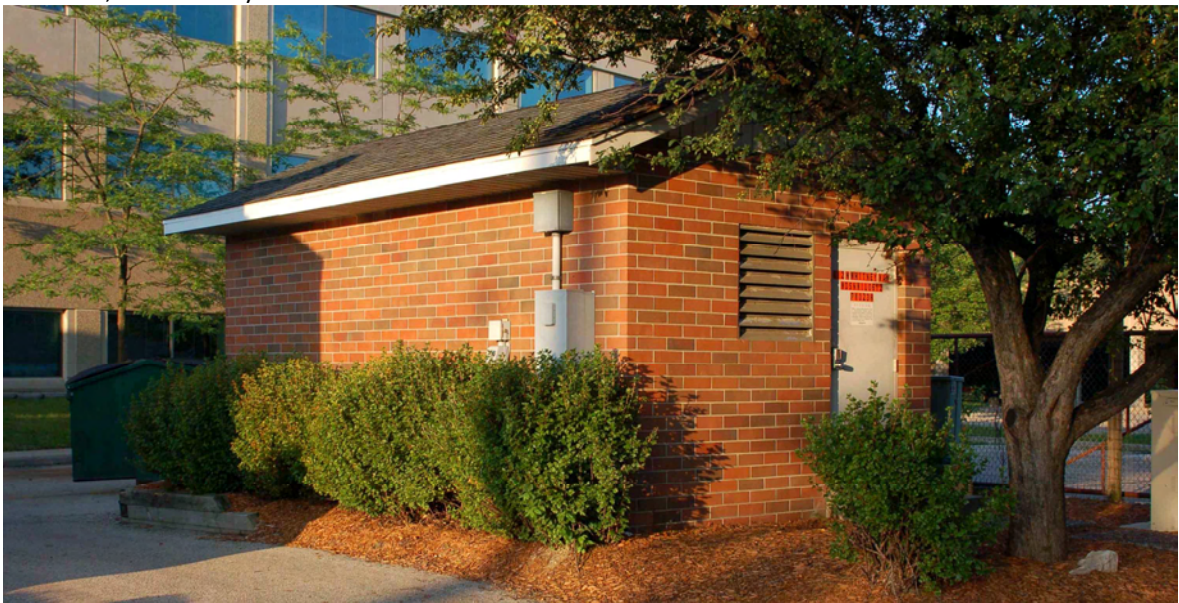
Easement, "AT+T Utility Shed"
