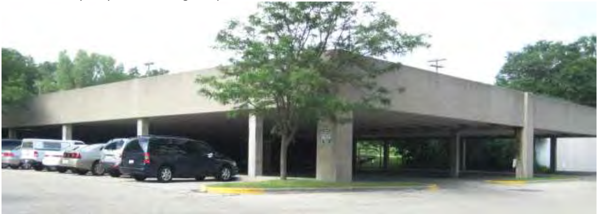
610 N. Whitney Way, "PSC Parking Ramp"
