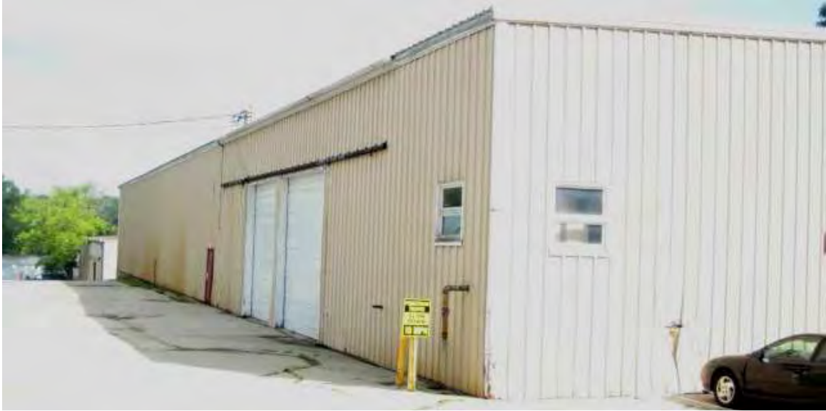
5115 University Avenue, "Upper Warehouse"
