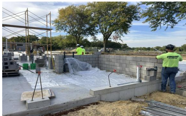
2 Masonry construction at Imagination Center site.
